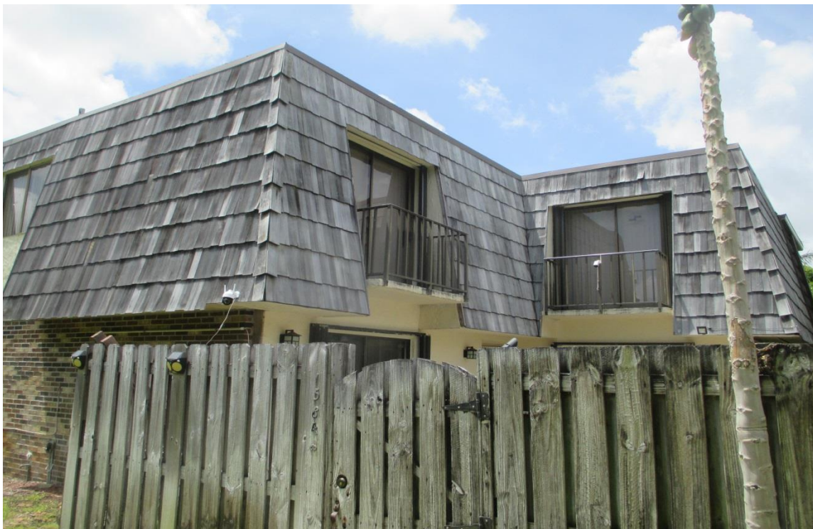
Mansard Roof Inspection Performed on Building #1584 at Forest Lakes - Unit: C – West Palm Beach, Fl.
