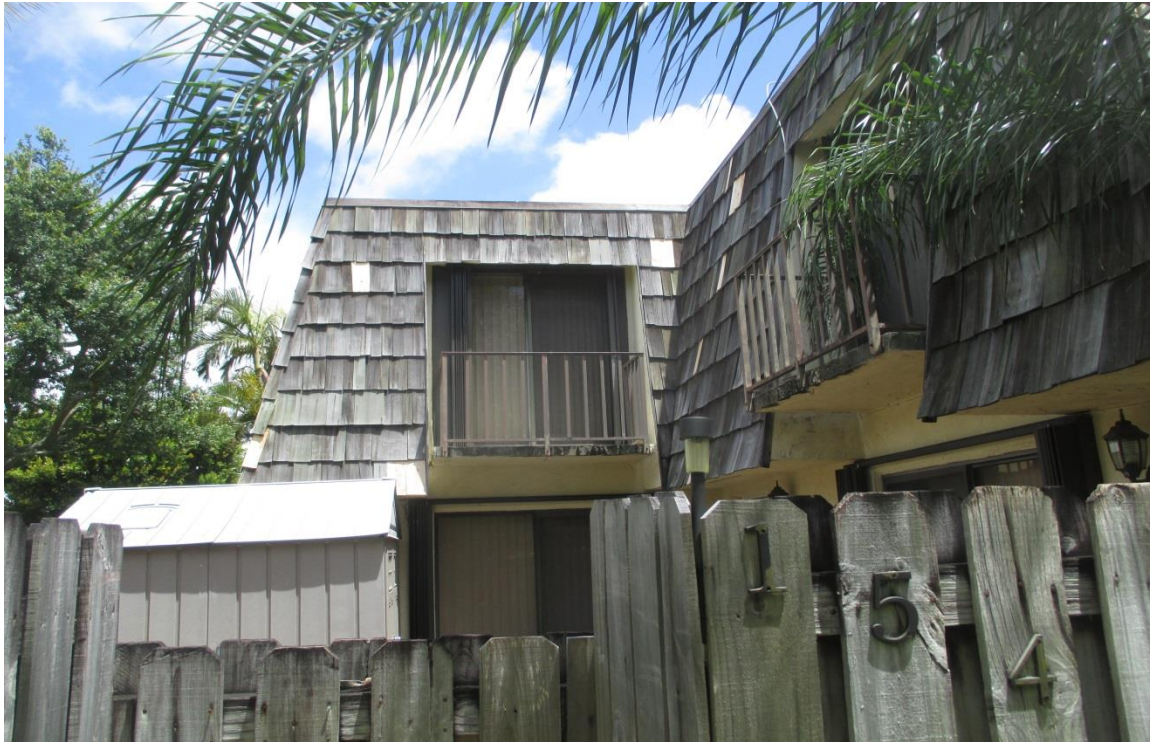
Mansard Roof Inspection Performed on Building #1545 at Forest Lakes - Unit: A – West Palm Beach, Fl.
