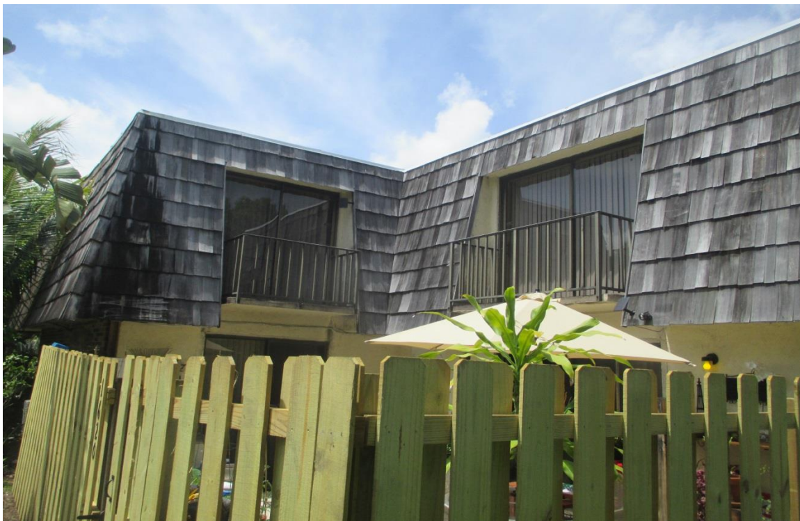
Mansard Roof Inspection Performed on Building #1620 at Forest Lakes - Unit: B – West Palm Beach, Fl.
