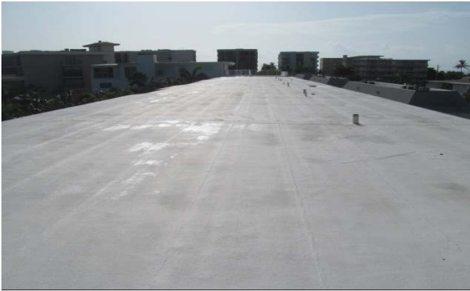
BUILT-UP ROOF COVERING
