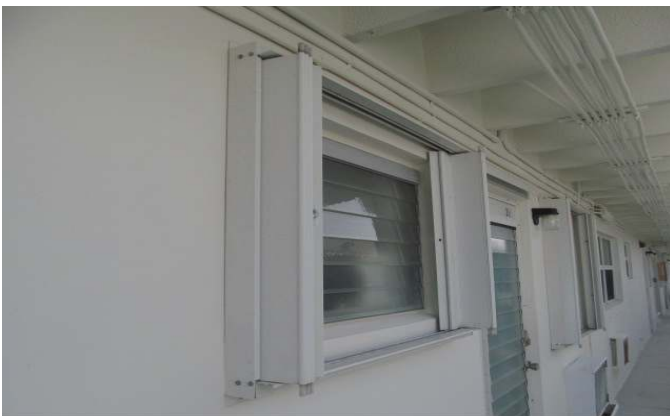
PROTECTED WITH RATED SHUTTERS
