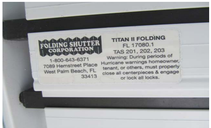
PROTECTED WITH RATED SHUTTERS
