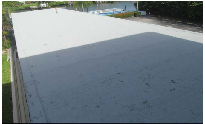
BUILT-UP ROOF COVERING
