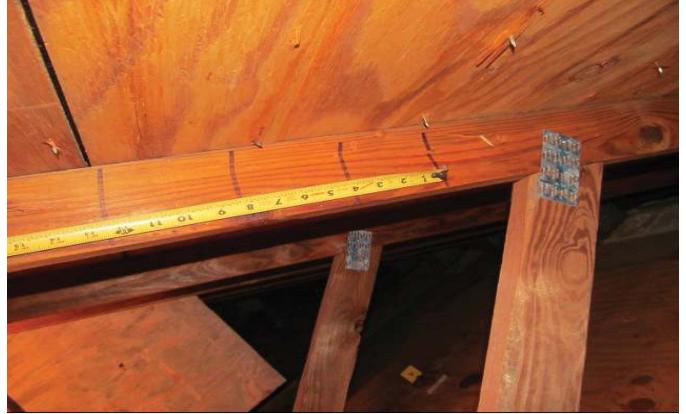
NAILS SPACED 6" ON THE EDGE
