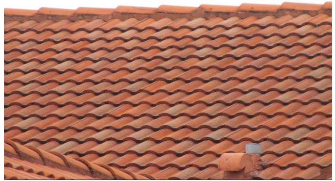
TILE ROOF COVERING
