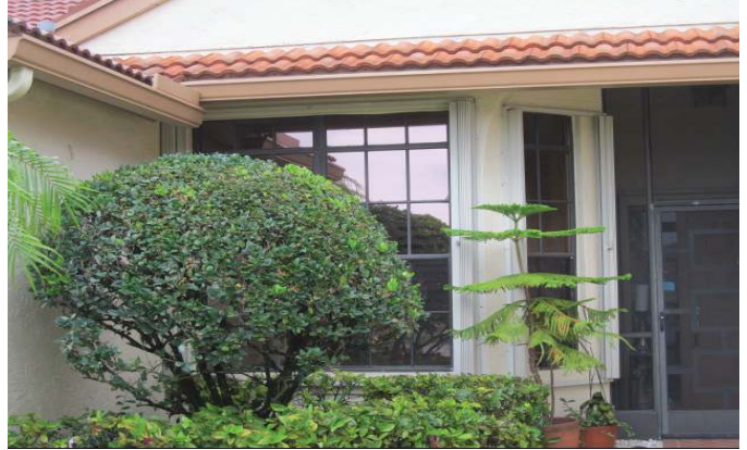
PROTECTED WITH UNVERIFIED SHUTTERS
