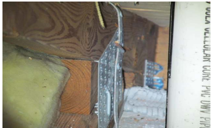
ANCHOR SIDE OF METAL CONNECTOR WITH 2 NAILS
