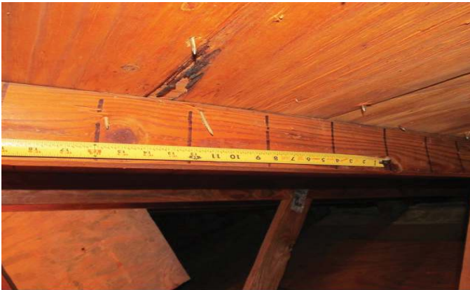
NAILS SPACED 6" IN THE FIELD
