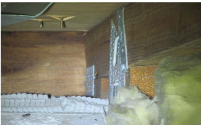
OPPOSING SIDE OF METAL CONNECTOR WITH 1 NAIL
