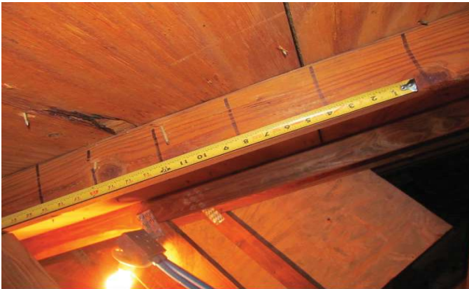
NAILS SPACED 6" IN THE FIELD
