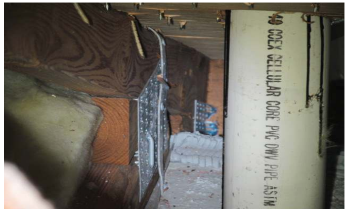
ANCHOR SIDE OF METAL CONNECTOR WITH 2 NAILS
