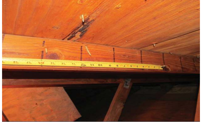
NAILS SPACED 6" ON THE EDGE
