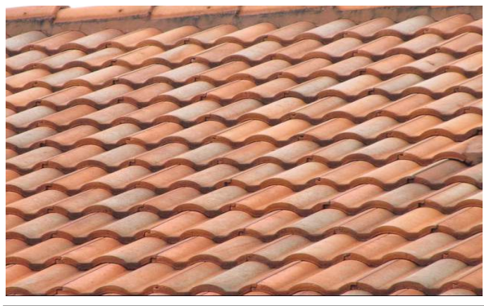
TILE ROOF COVERING
