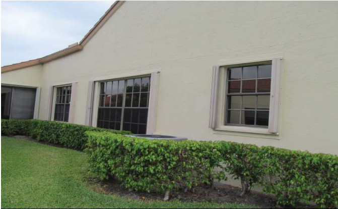
PROTECTED WITH UNVERIFIED SHUTTERS
