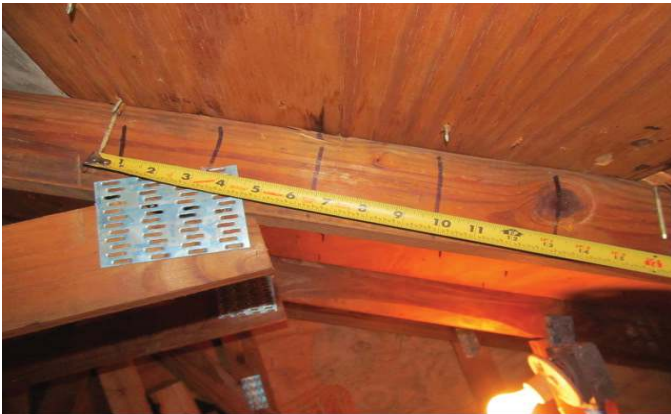
NAILS SPACED 6" IN THE FIELD
