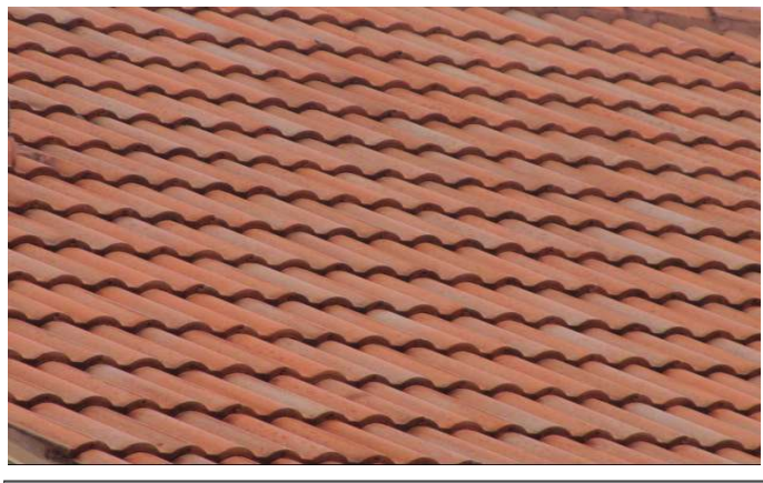
TILE ROOF COVERING
