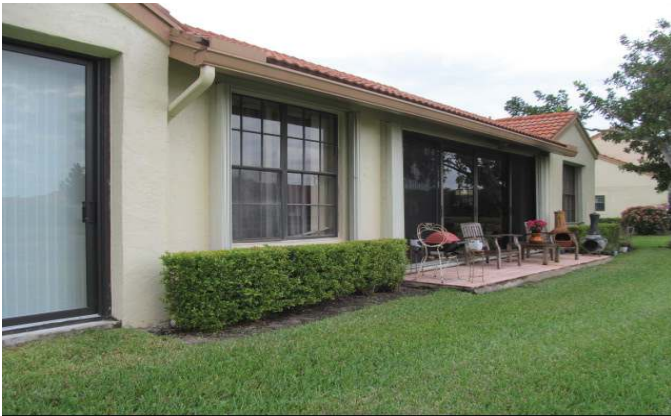
PROTECTED WITH UNVERIFIED SHUTTERS
