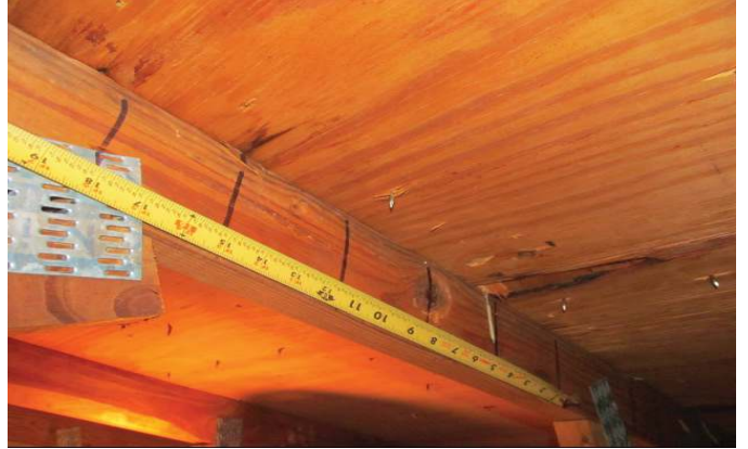
NAILS SPACED 6" ON THE EDGE
