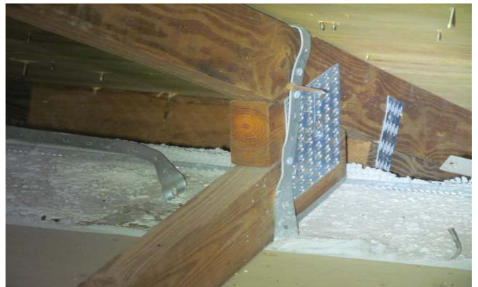
ANCHOR SIDE OF METAL CONNECTOR WITH 2 NAILS
