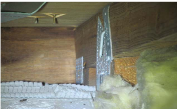
OPPOSING SIDE OF METAL CONNECTOR WITH 1 NAIL
