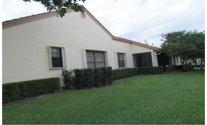
PROTECTED WITH UNVERIFIED SHUTTERS
