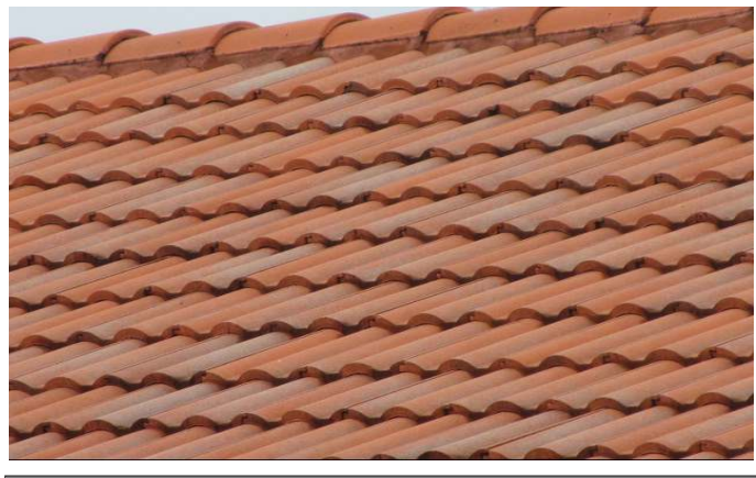
TILE ROOF COVERING
