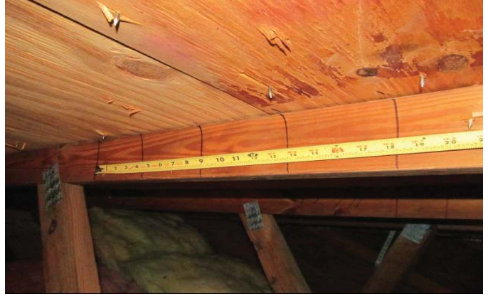
NAILS SPACED 6" ON THE EDGE
