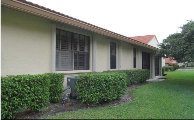
PROTECTED WITH UNVERIFIED SHUTTERS
