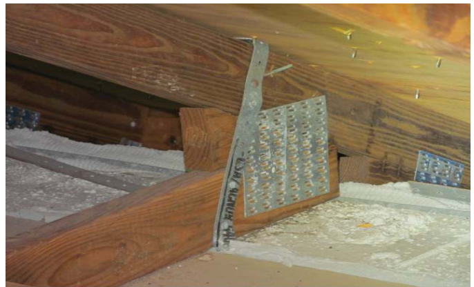
ANCHOR SIDE OF METAL CONNECTOR WITH 2 NAILS
