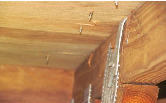
OPPOSING SIDE OF METAL CONNECTOR WITH 1 NAIL
