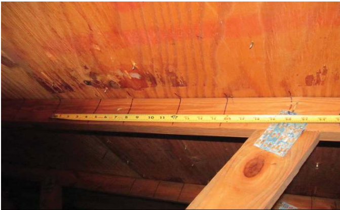
NAILS SPACED 6" IN THE FIELD
