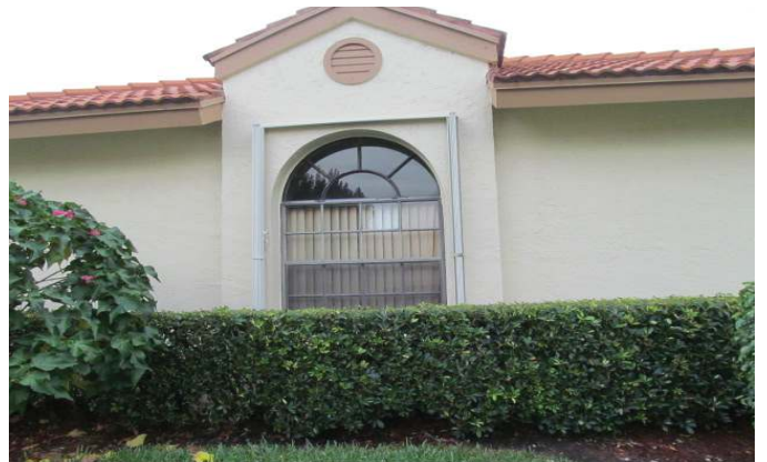
PROTECTED WITH UNVERIFIED SHUTTERS
