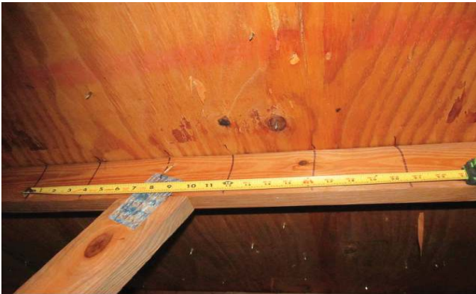
NAILS SPACED 6" IN THE FIELD
