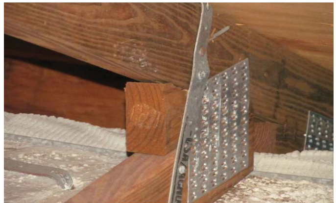
ANCHOR SIDE OF METAL CONNECTOR WITH 2 NAILS
