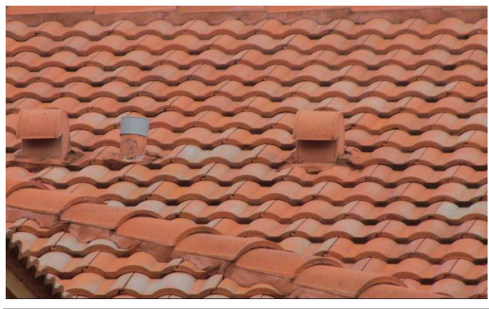
TILE ROOF COVERING
