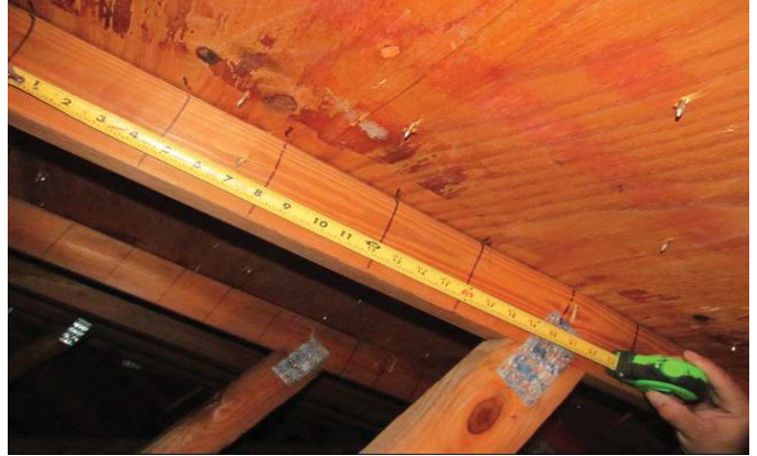
NAILS SPACED 6" ON THE EDGE
