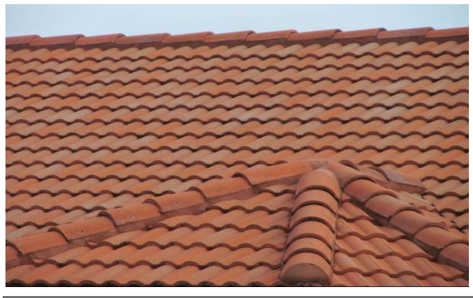
TILE ROOF COVERING
