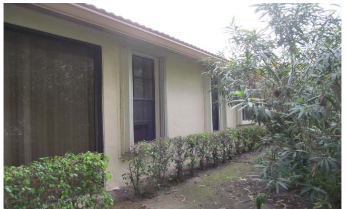
PROTECTED WITH UNVERIFIED SHUTTERS
