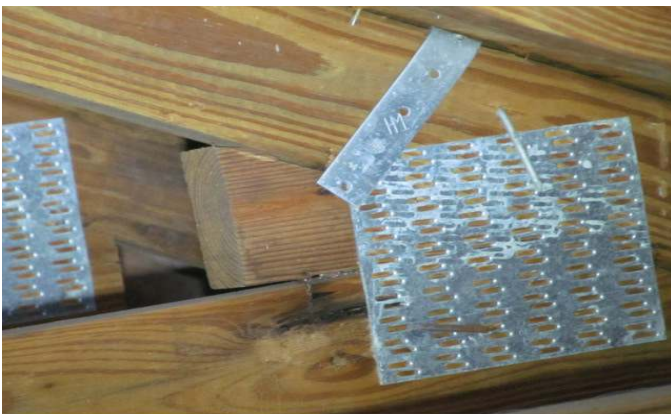
OPPOSING SIDE OF METAL CONNECTOR WITH 1 NAIL
