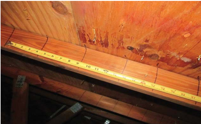
NAILS SPACED 6" IN THE FIELD
