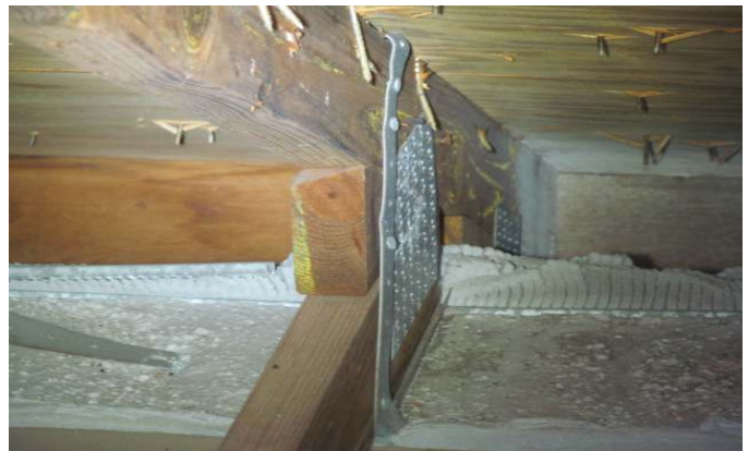
ANCHOR SIDE OF METAL CONNECTOR WITH 2 NAILS
