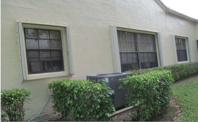
PROTECTED WITH UNVERIFIED SHUTTERS
