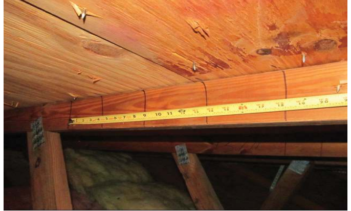
NAILS SPACED 6" ON THE EDGE
