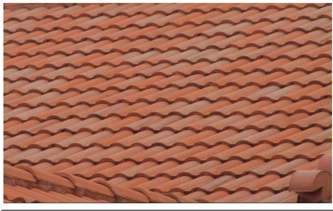
TILE ROOF COVERING
