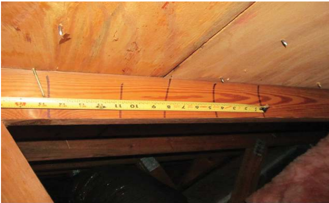
NAILS SPACED 6" IN THE FIELD
