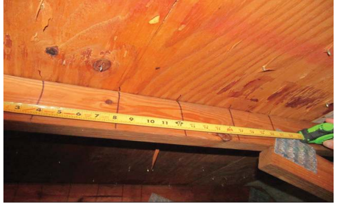
NAILS SPACED 6" ON THE EDGE
