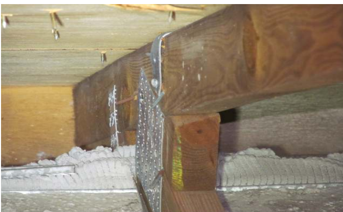
OPPOSING SIDE OF METAL CONNECTOR WITH 1 NAIL
