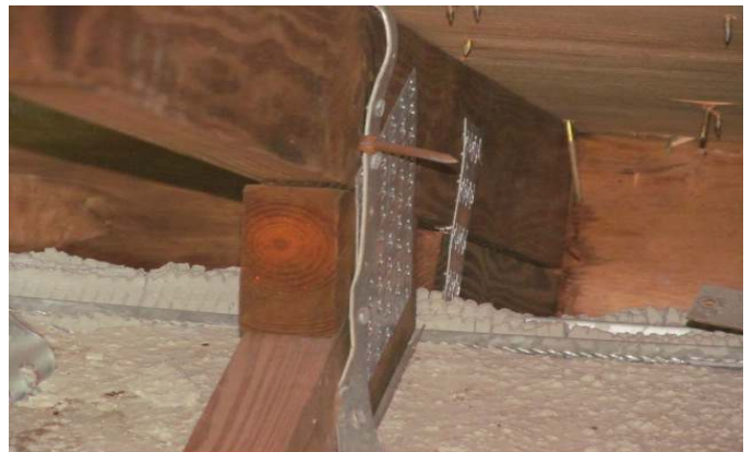
ANCHOR SIDE OF METAL CONNECTOR WITH 2 NAILS
