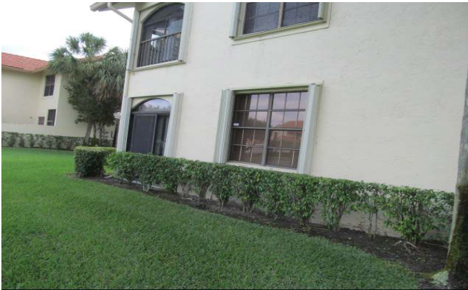
PROTECTED WITH UNVERIFIED SHUTTERS
