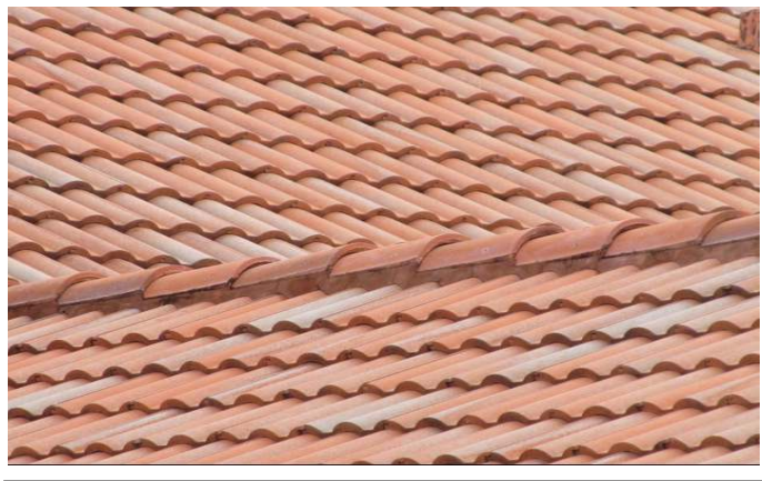
TILE ROOF COVERING
