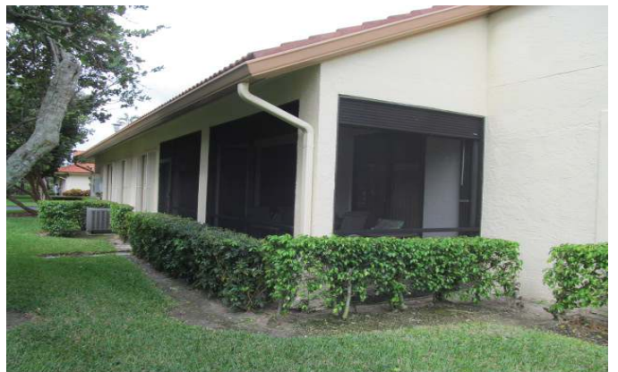
PROTECTED WITH UNVERIFIED SHUTTERS
