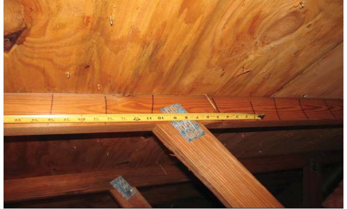
NAILS SPACED 6" ON THE EDGE
