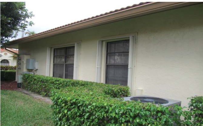
PROTECTED WITH UNVERIFIED SHUTTERS
