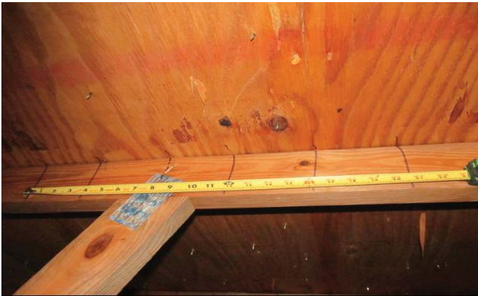
NAILS SPACED 6" IN THE FIELD
