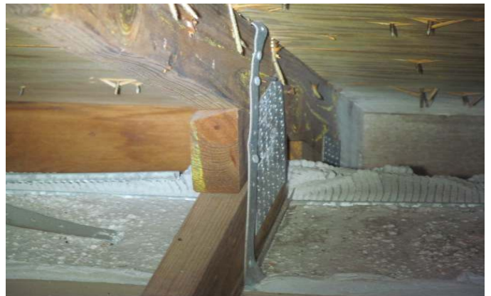
ANCHOR SIDE OF METAL CONNECTOR WITH 2 NAILS
