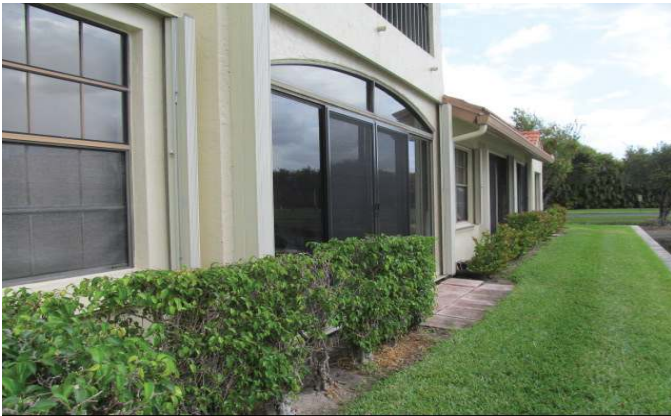
PROTECTED WITH UNVERIFIED SHUTTERS
