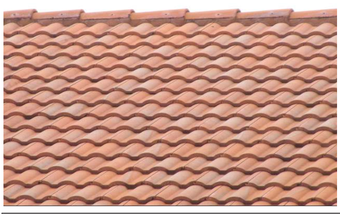
TILE ROOF COVERING
