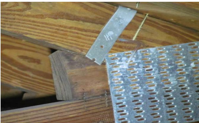
OPPOSING SIDE OF METAL CONNECTOR WITH 1 NAIL
