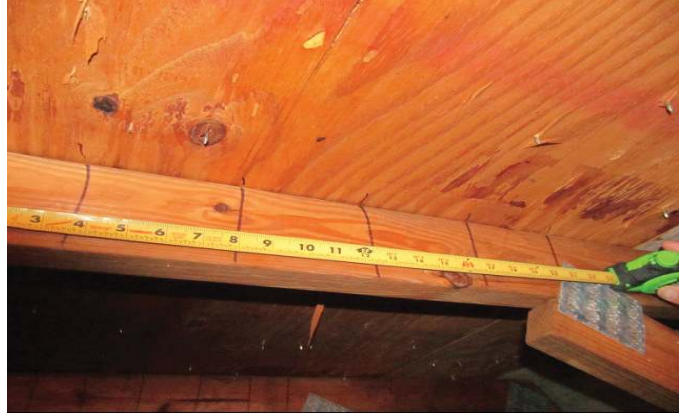
NAILS SPACED 6" ON THE EDGE
