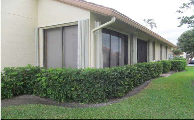
PROTECTED WITH UNVERIFIED SHUTTERS
