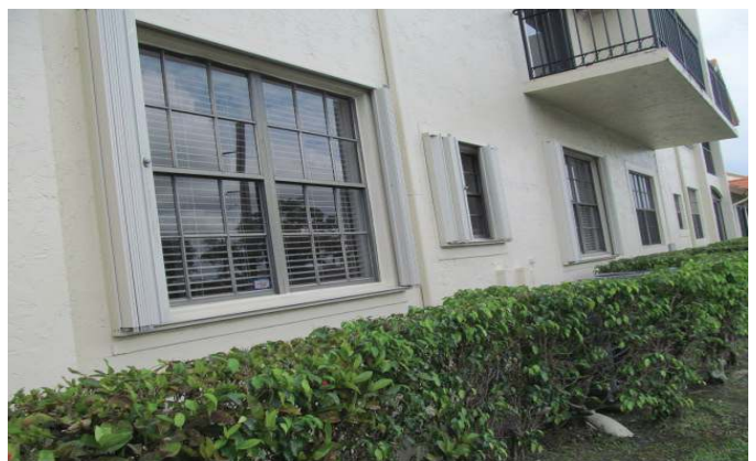
PROTECTED WITH UNVERIFIED SHUTTERS
