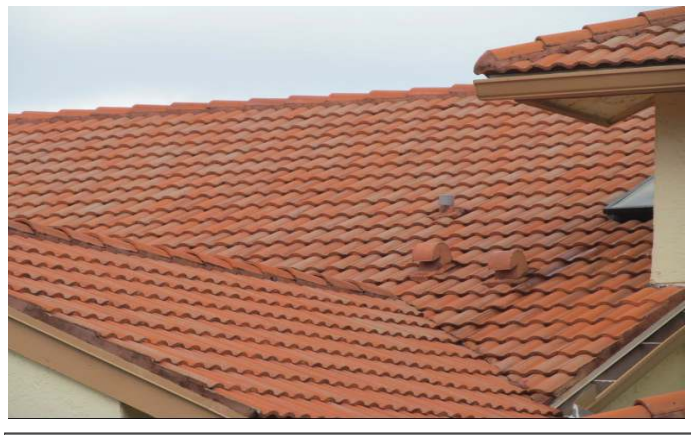
TILE ROOF COVERING
