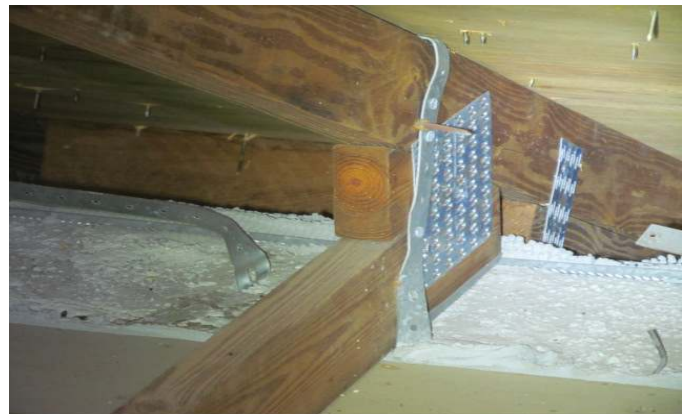
ANCHOR SIDE OF METAL CONNECTOR WITH 2 NAILS
