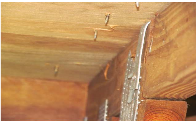
OPPOSING SIDE OF METAL CONNECTOR WITH 1 NAIL
