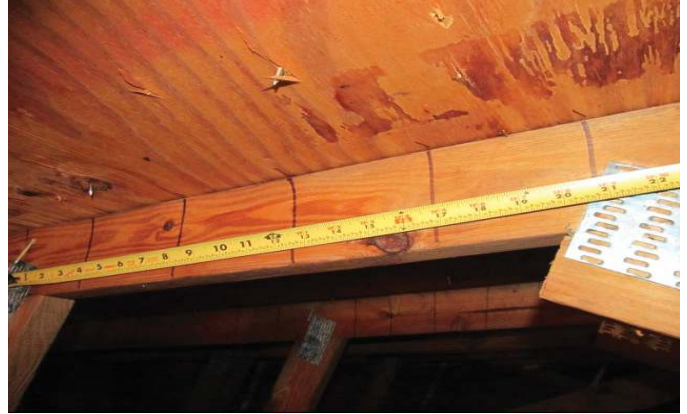
NAILS SPACED 6" ON THE EDGE
