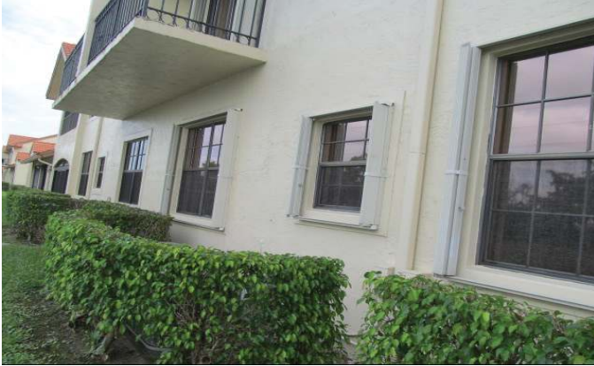
PROTECTED WITH UNVERIFIED SHUTTERS
