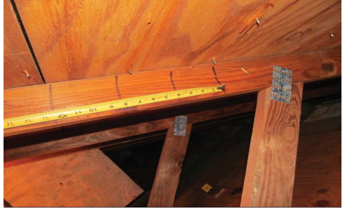
NAILS SPACED 6" ON THE EDGE
