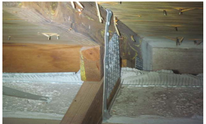
ANCHOR SIDE OF METAL CONNECTOR WITH 2 NAILS
