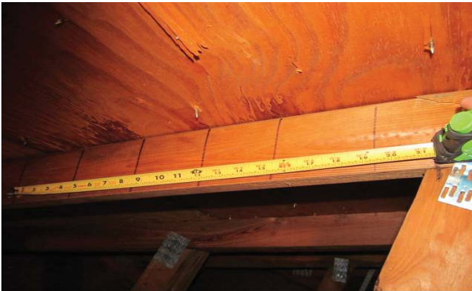
NAILS SPACED 6" IN THE FIELD
