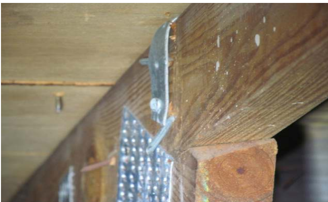
OPPOSING SIDE OF METAL CONNECTOR WITH 1 NAIL
