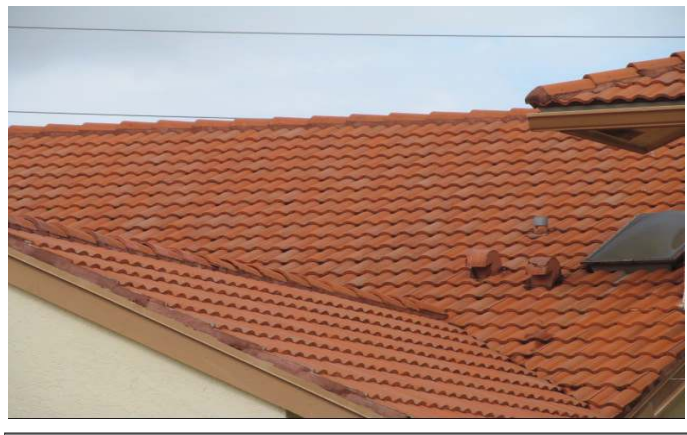
TILE ROOF COVERING
