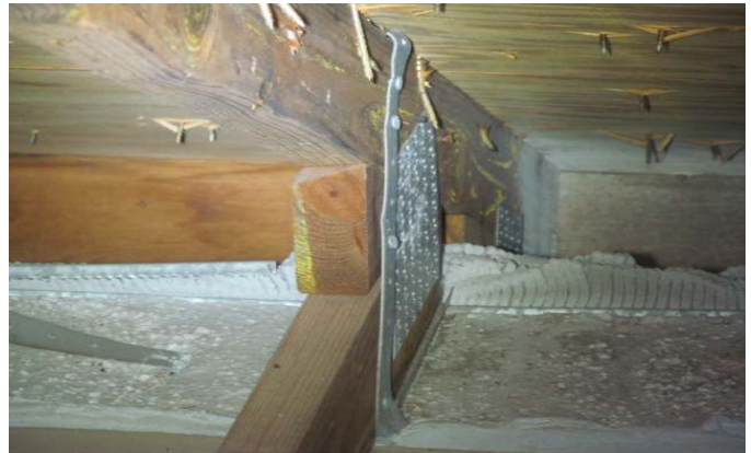
ANCHOR SIDE OF METAL CONNECTOR WITH 2 NAILS
