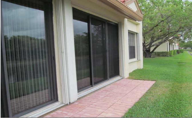
PROTECTED WITH UNVERIFIED SHUTTERS
