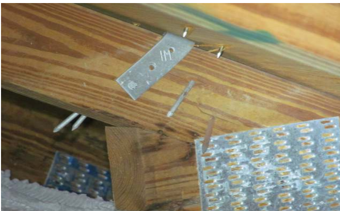
OPPOSING SIDE OF METAL CONNECTOR WITH 1 NAIL
