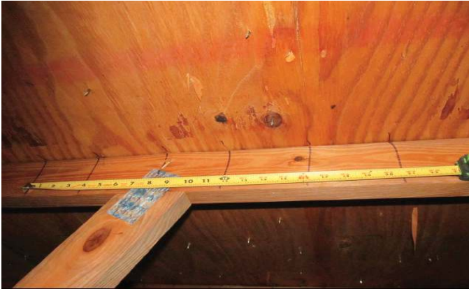
NAILS SPACED 6" IN THE FIELD
