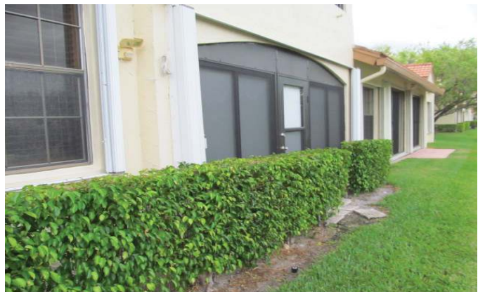
PROTECTED WITH UNVERIFIED SHUTTERS
