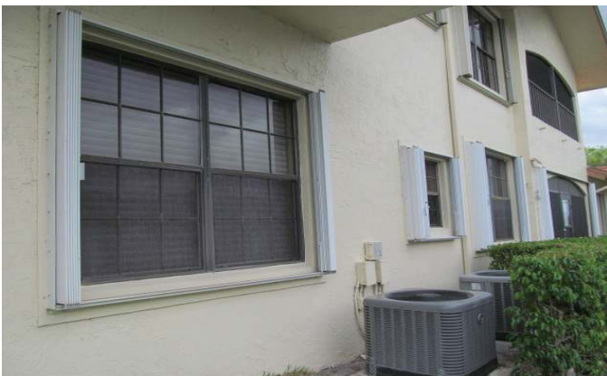
PROTECTED WITH UNVERIFIED SHUTTERS
