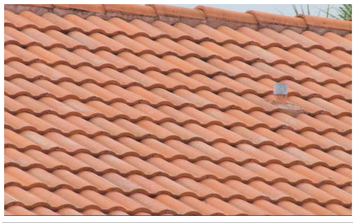
TILE ROOF COVERING
