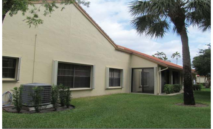
PROTECTED WITH UNVERIFIED SHUTTERS
