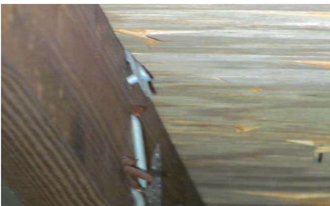
OPPOSING SIDE OF METAL CONNECTOR WITH 1 NAIL
