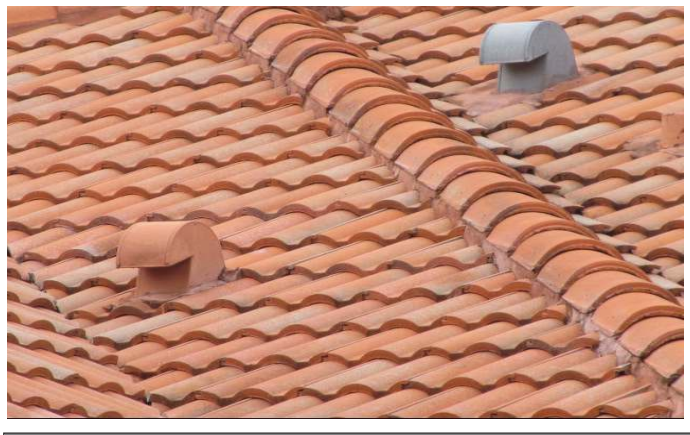
TILE ROOF COVERING
