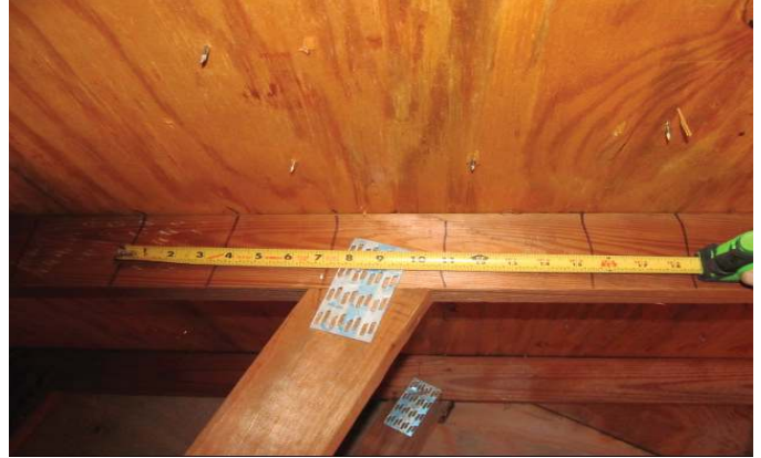
NAILS SPACED 6" ON THE EDGE
