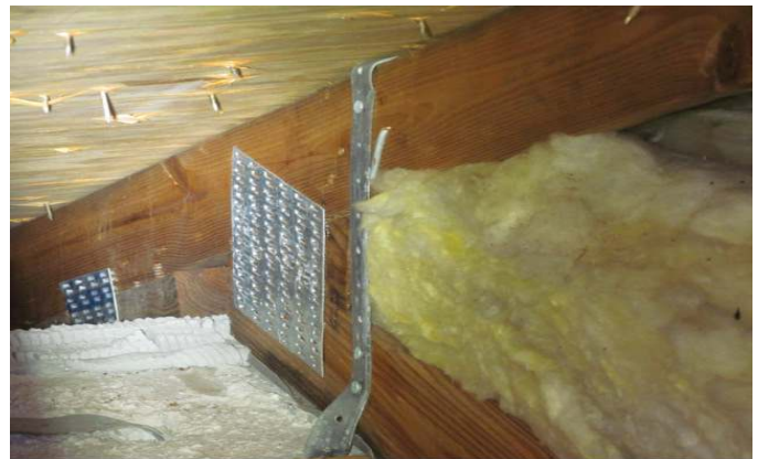
ANCHOR SIDE OF METAL CONNECTOR WITH 2 NAILS
