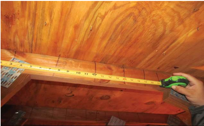
NAILS SPACED 6" IN THE FIELD
