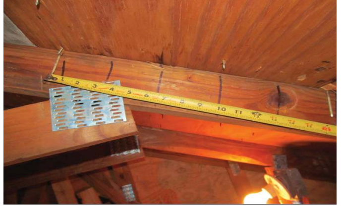
NAILS SPACED 6" ON THE EDGE
