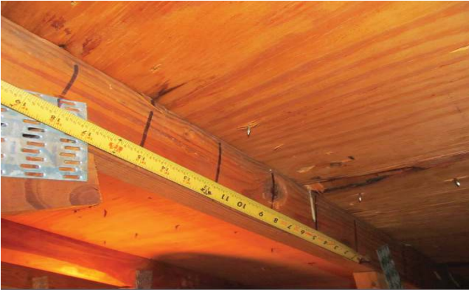
NAILS SPACED 6" IN THE FIELD
