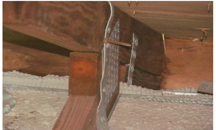
ANCHOR SIDE OF METAL CONNECTOR WITH 2 NAILS
