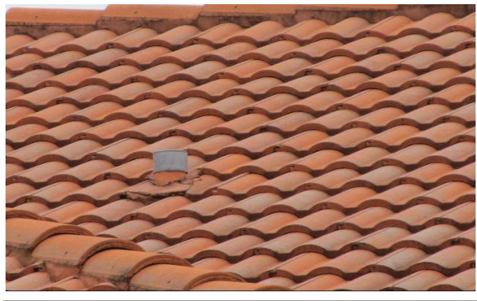
TILE ROOF COVERING
