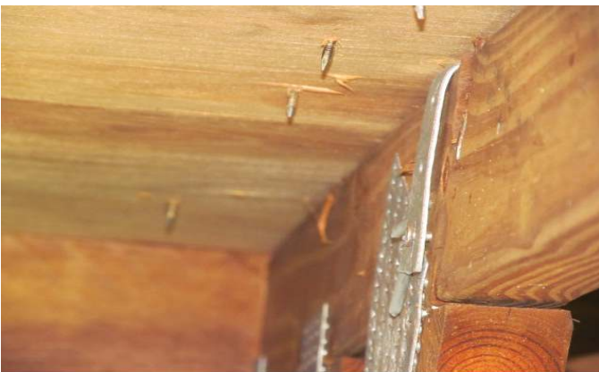
OPPOSING SIDE OF METAL CONNECTOR WITH 1 NAIL
