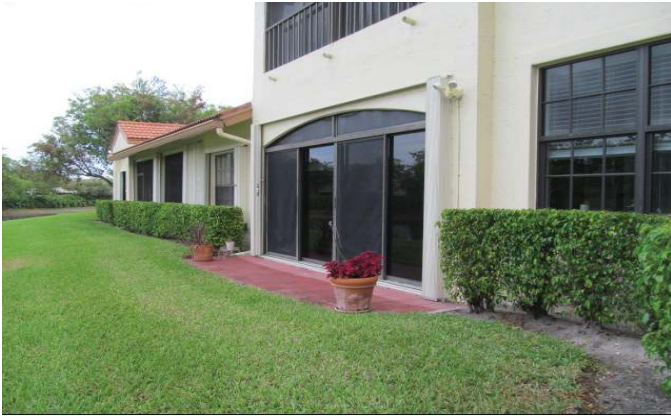
PROTECTED WITH UNVERIFIED SHUTTERS
