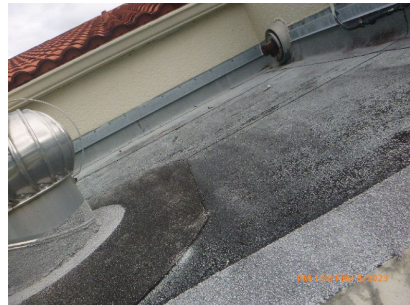
Built Up/Rolled Asphalt (Flat) Roof Covering
