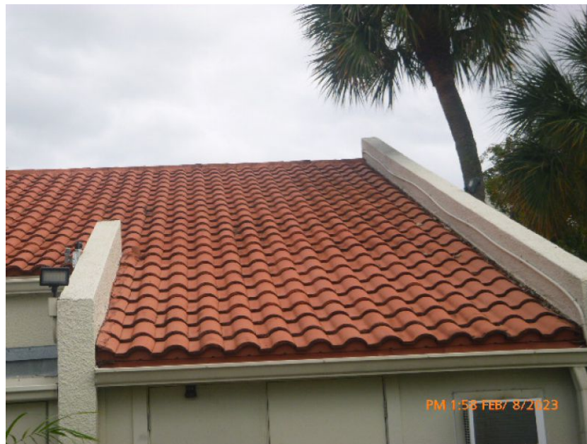
Concrete/Clay Tile Roof Covering
