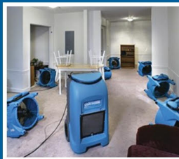
Structural Drying
