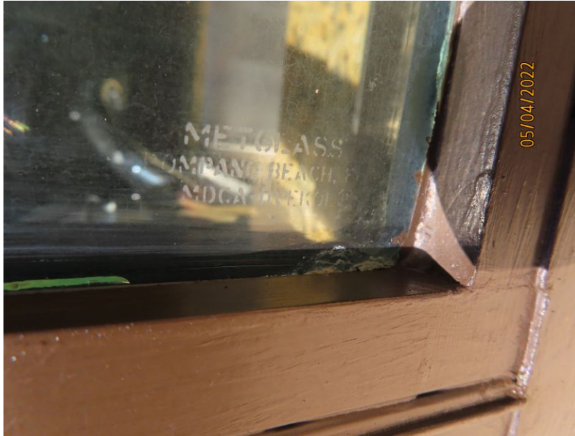
Impact Rated Glazed Door Etching/Engraving
