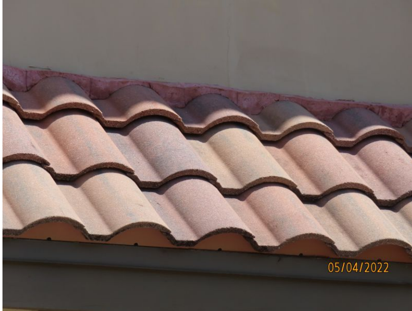
Concrete/Clay Tile Roof Covering
