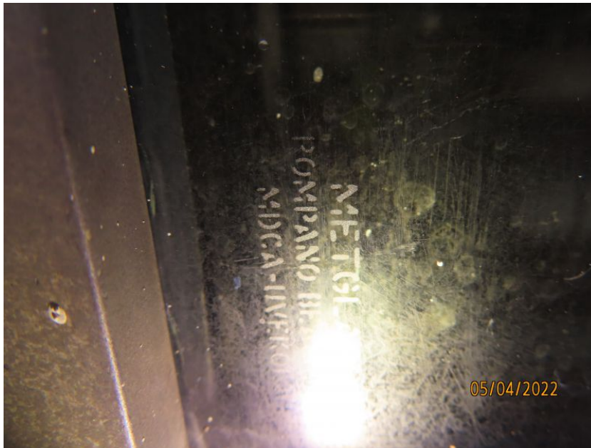
Impact Rated Glass Window Etching/Engraving
