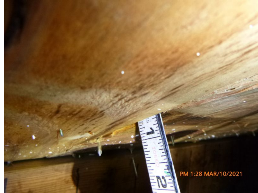
19/32" Deck Thickness Confirmed
