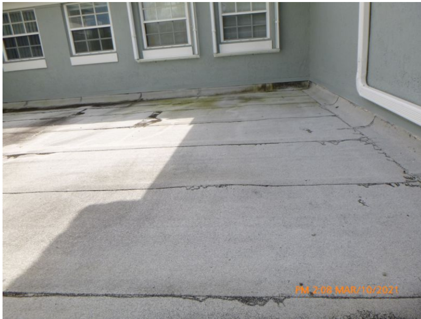
Built-Up/Rolled Asphalt Roof Covering
