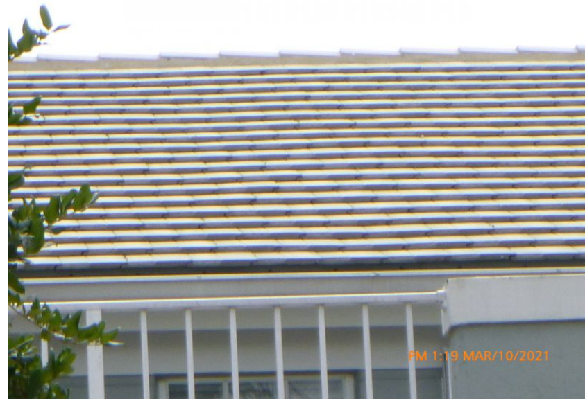
Concrete/Clay Tile Roof Covering
