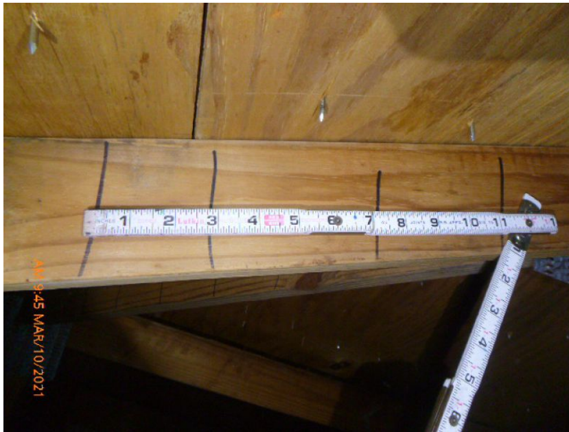
8d Nails or Greater in Size Spaced 6" in the Field
