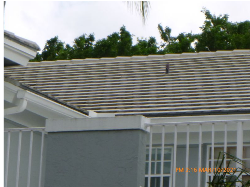
Concrete/Clay Tile Roof Covering
