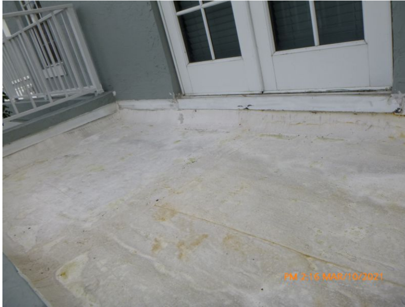
Built-Up/Rolled Asphalt Roof Covering
