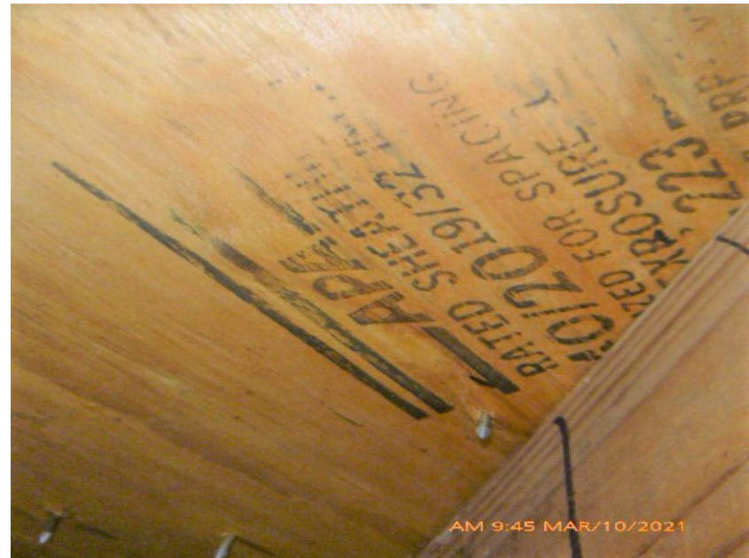
19/32" Deck Thickness Confirmed
