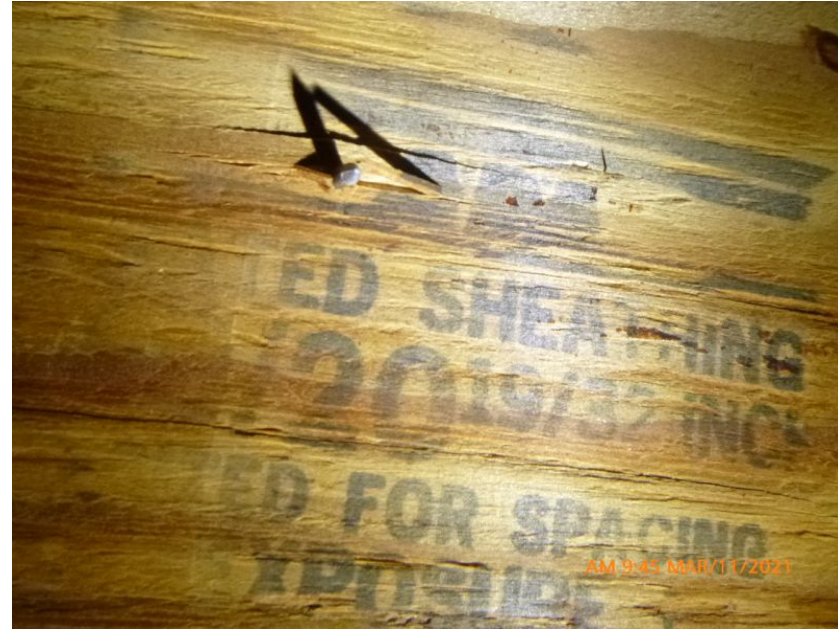
19/32" Deck Thickness Confirmed
