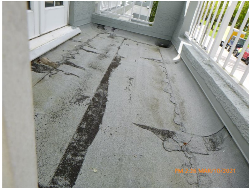
Built-Up/Rolled Asphalt Roof Covering
