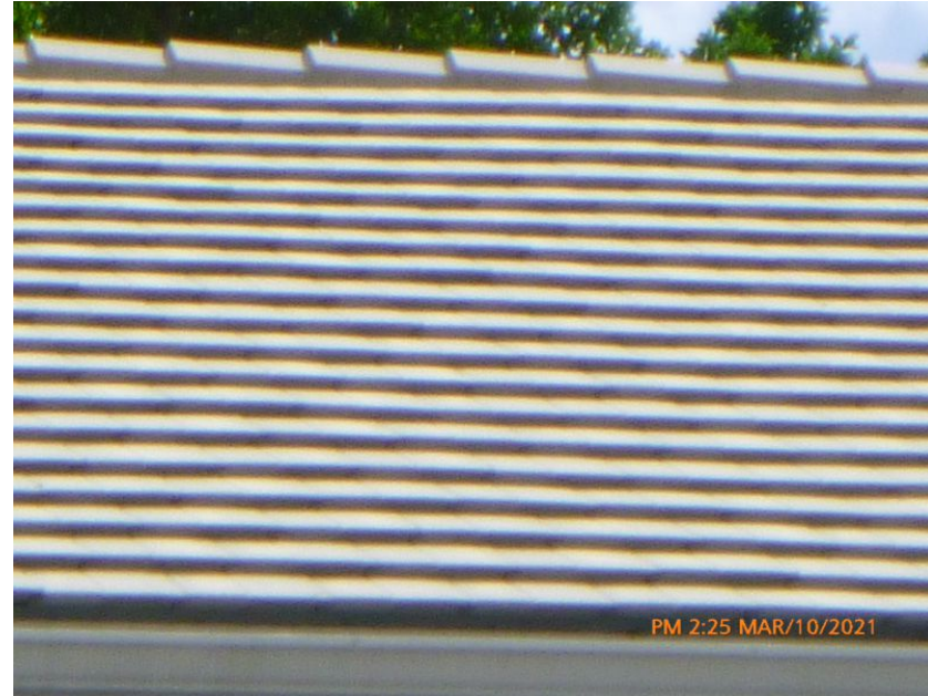
Concrete/Clay Tile Roof Covering
