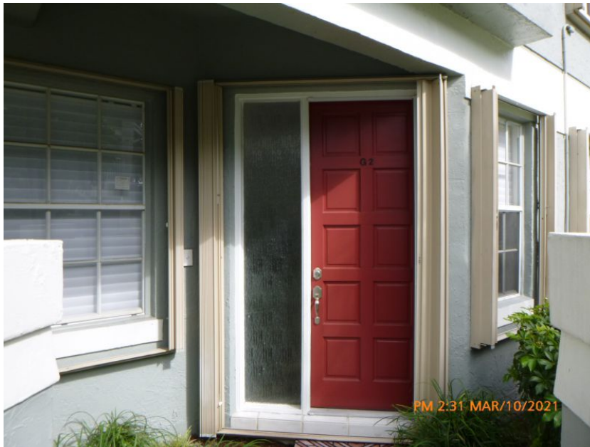
Accordion Shutter - Unverified as Impact
