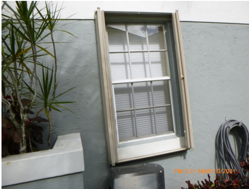
Accordion Shutter - Unverified as Impact
