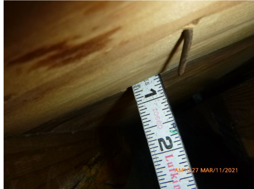
19/32" Deck Thickness Confirmed
