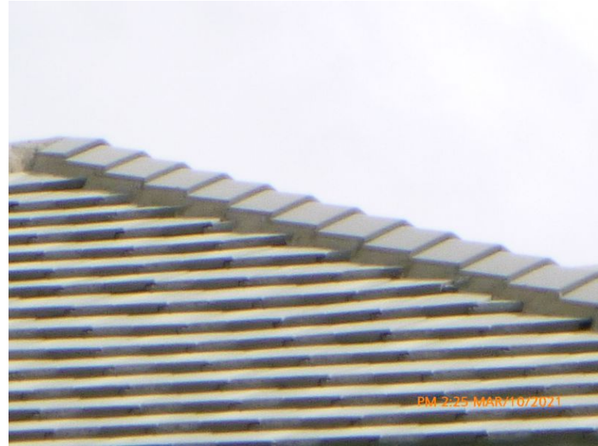
Concrete/Clay Tile Roof Covering
