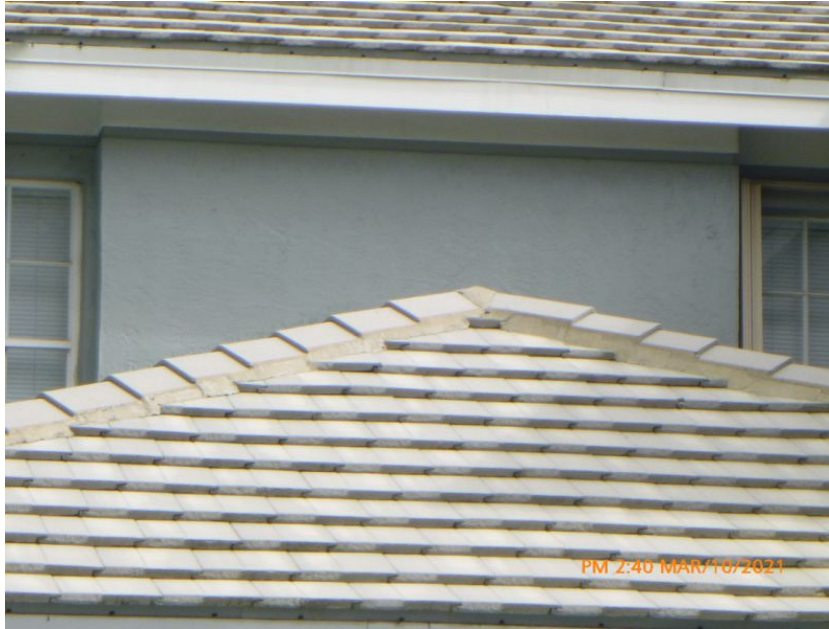
Concrete/Clay Tile Roof Covering
