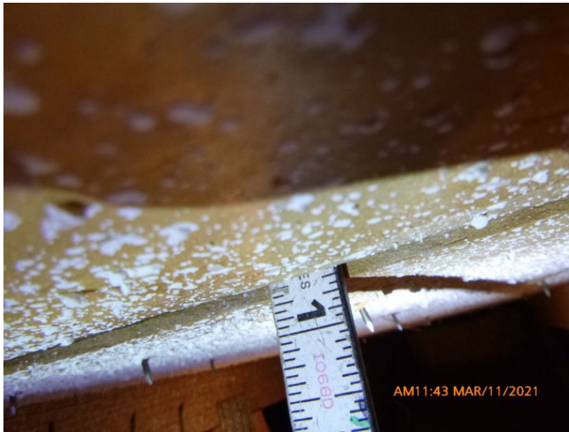
19/32" Deck Thickness Confirmed
