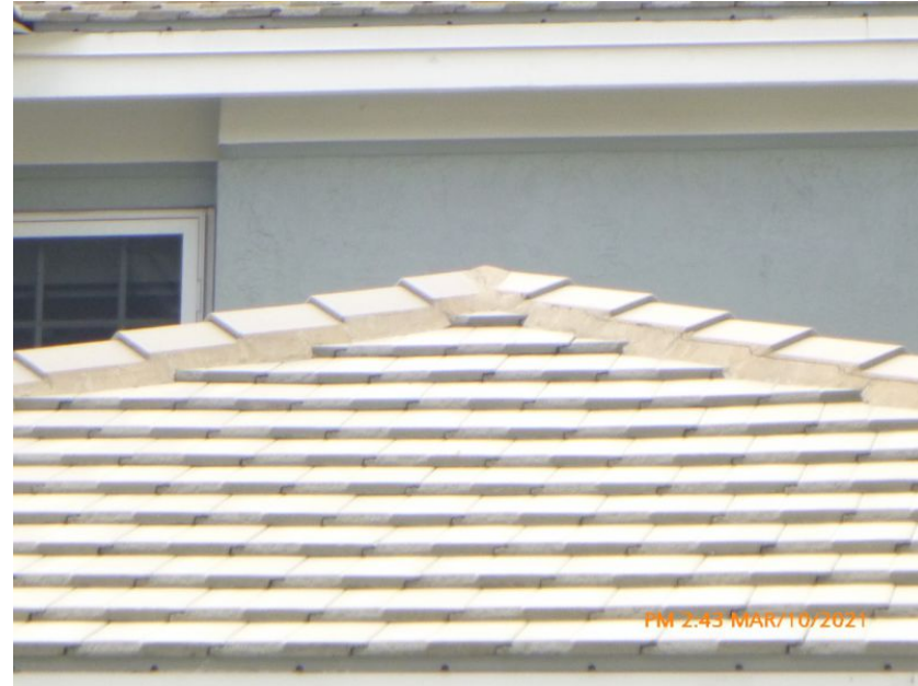
Concrete/Clay Tile Roof Covering
