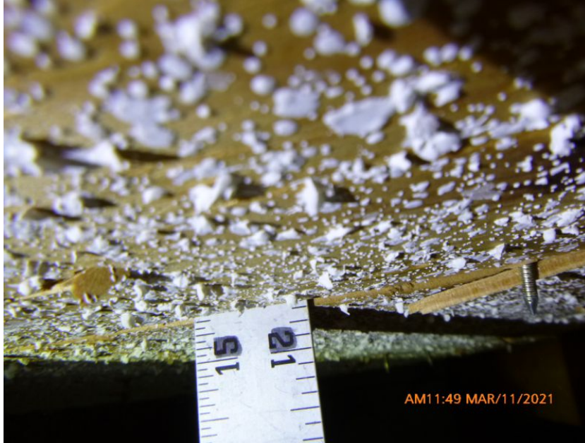
19/32" Deck Thickness Confirmed
