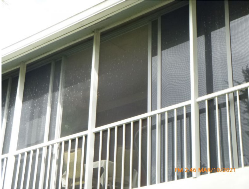
Unprotected Glazed Entry Door
