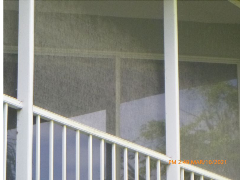
Unprotected Glazed Entry Door
