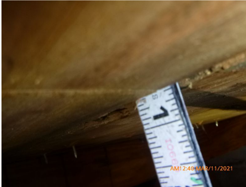
19/32" Deck Thickness Confirmed
