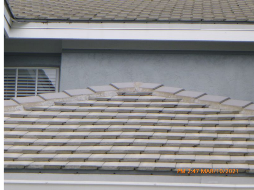
Concrete/Clay Tile Roof Covering
