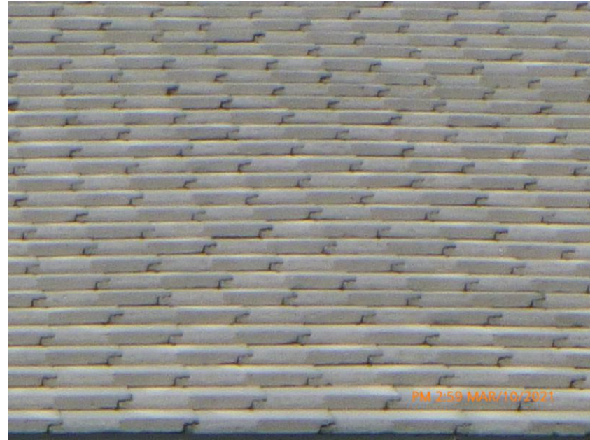
Concrete/Clay Tile Roof Covering
