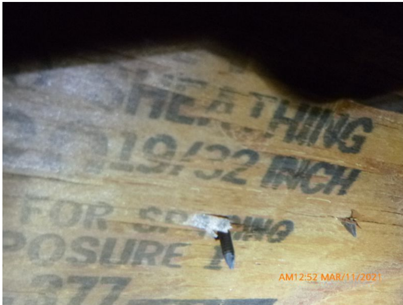
19/32" Deck Thickness Confirmed
