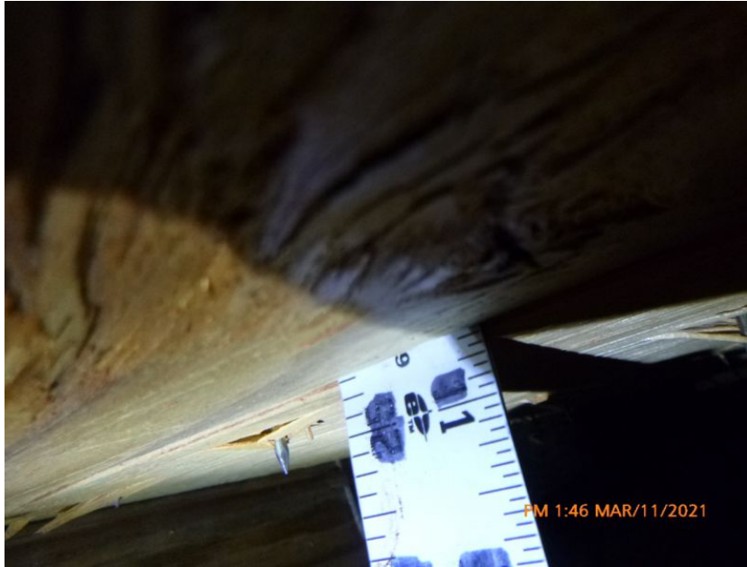
19/32" Deck Thickness Confirmed
