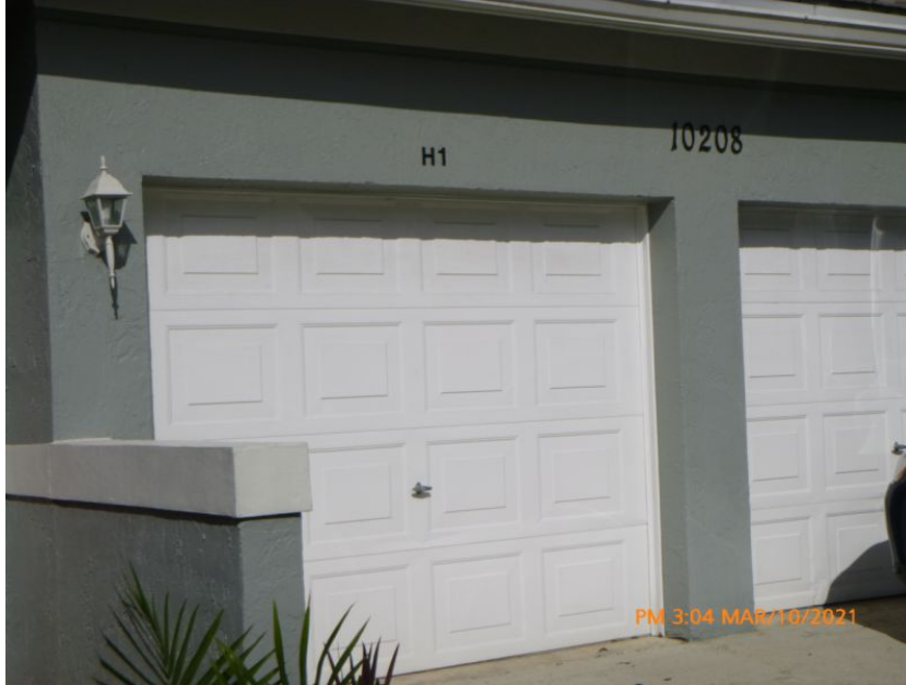
Unprotected Solid Garage Door
