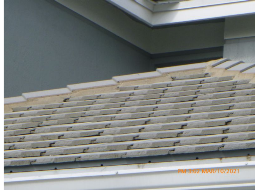
Concrete/Clay Tile Roof Covering
