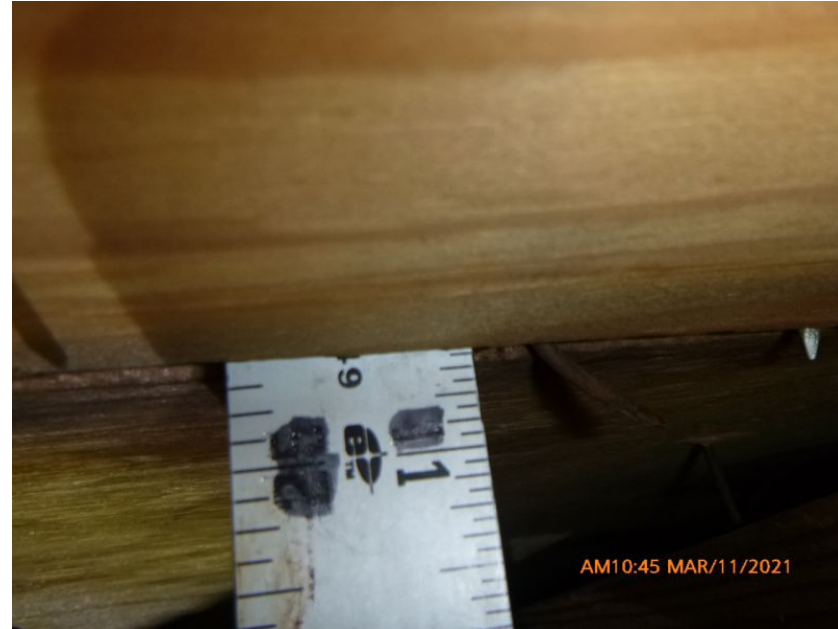
19/32" Deck Thickness Confirmed
