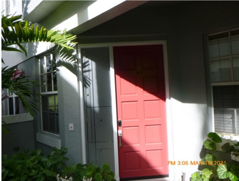
Unprotected Solid Entry Door
