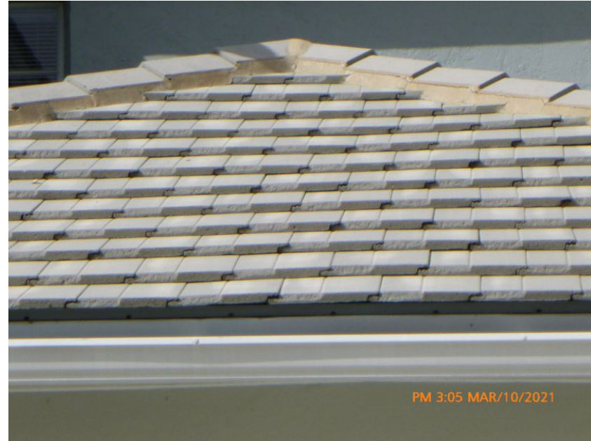
Concrete/Clay Tile Roof Covering
