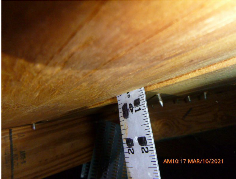
19/32" Deck Thickness Confirmed
