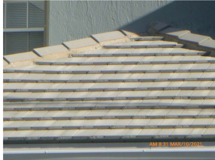
Concrete/Clay Tile Roof Covering
