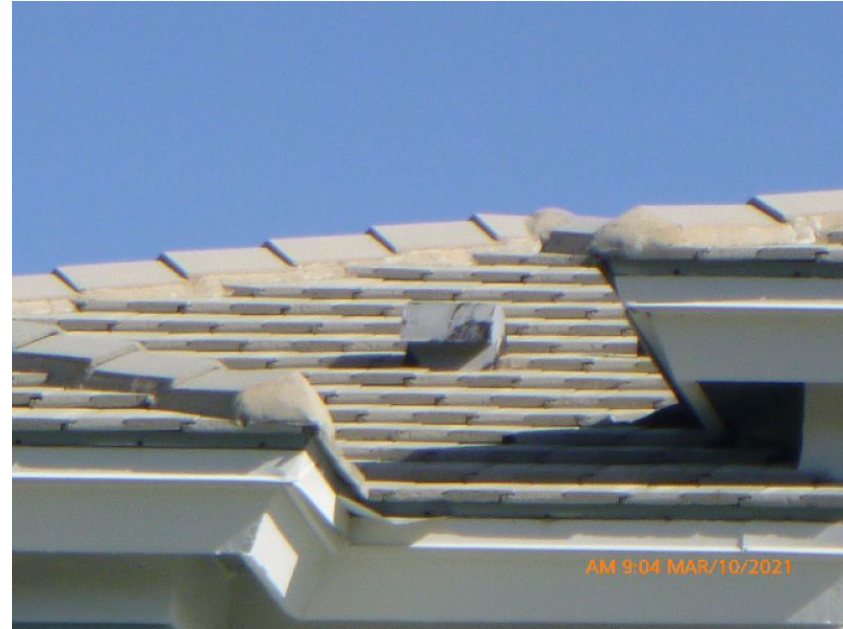
Concrete/Clay Tile Roof Covering
