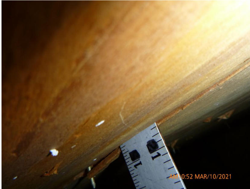
19/32" Deck Thickness Confirmed
