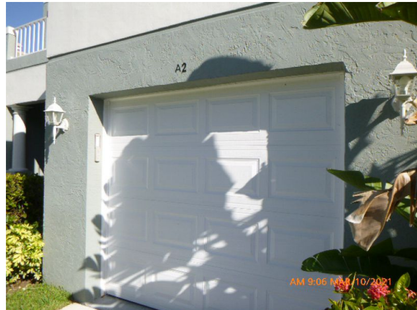
Unprotected Solid Garage Door
