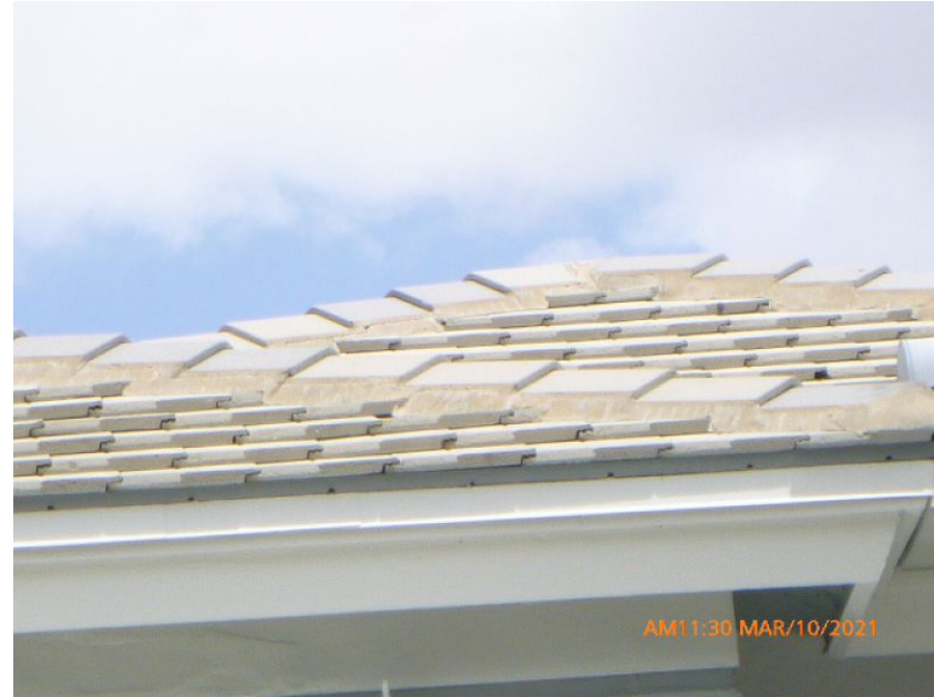
Concrete/Clay Tile Roof Covering
