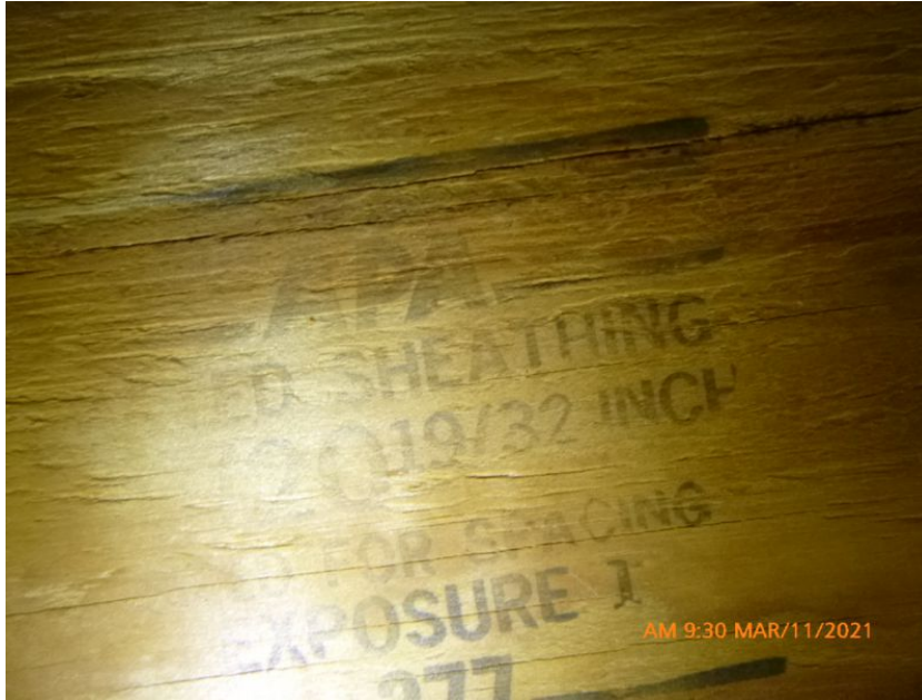
19/32" Deck Thickness Confirmed
