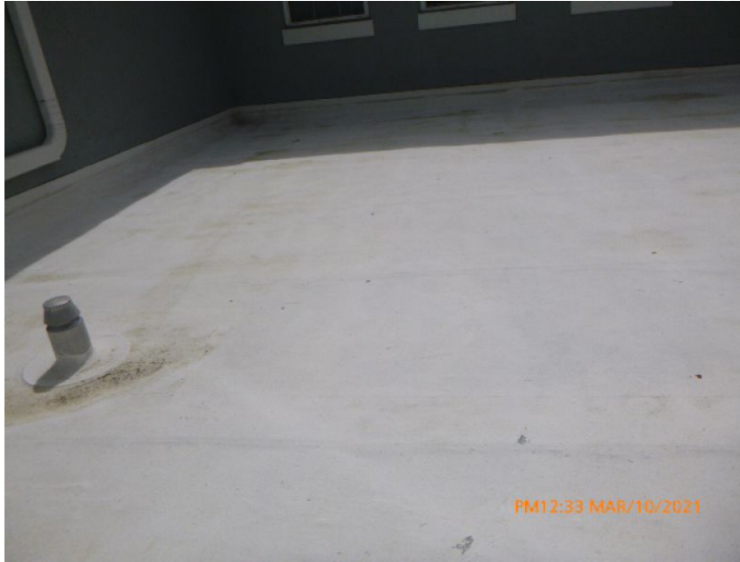
Built-Up/Rolled Asphalt Roof Covering
