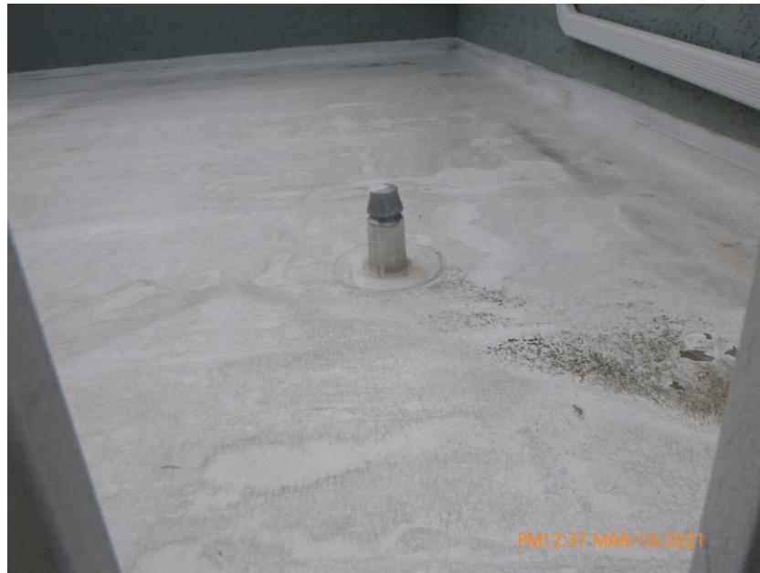
Built-Up/Rolled Asphalt Roof Covering
