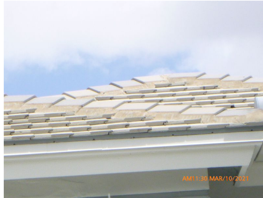
Concrete/Clay Tile Roof Covering
