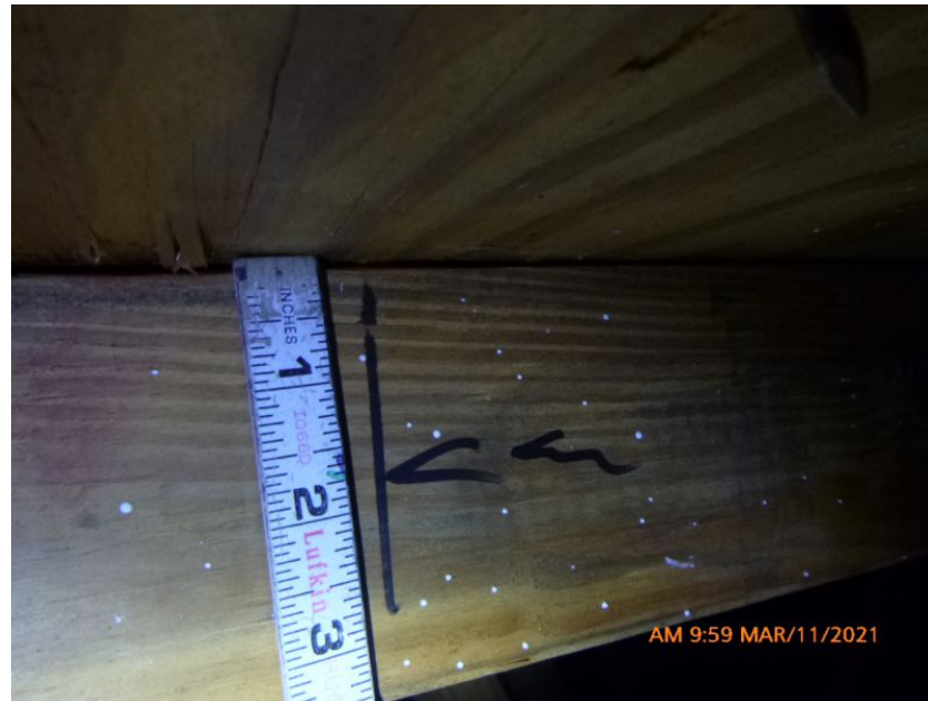
8d Nails; Measured with i520 Zircon Due to No Shiner
