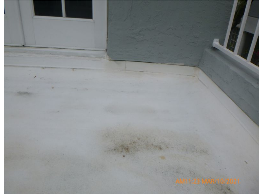
Built-Up/Rolled Asphalt Roof Covering
