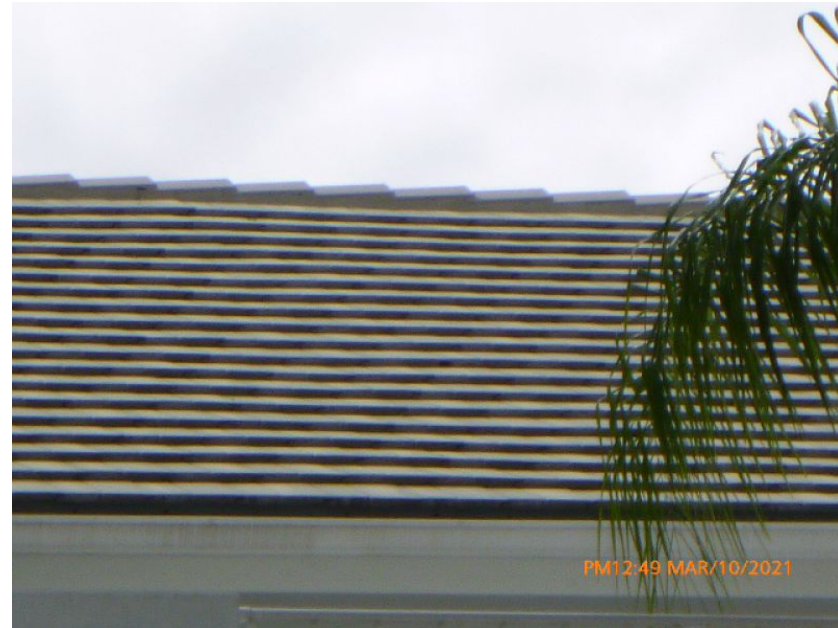
Concrete/Clay Tile Roof Covering
