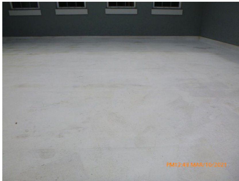
Built-Up/Rolled Asphalt Roof Covering
