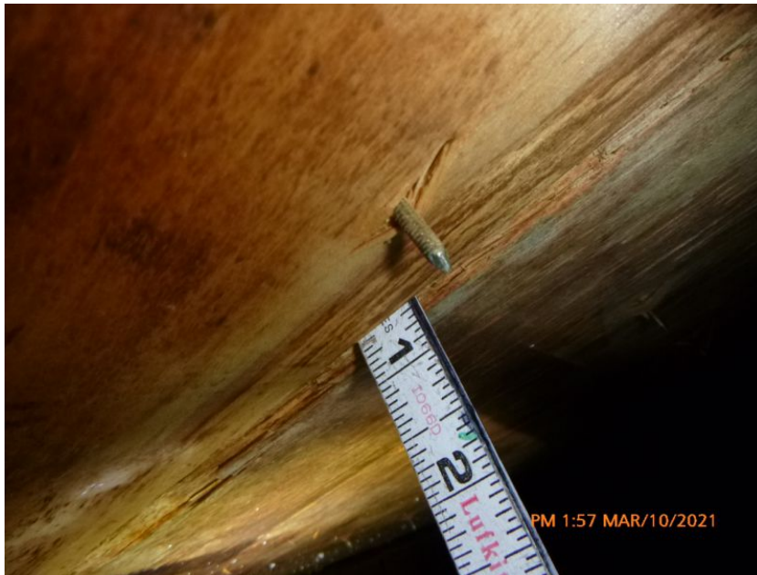
19/32" Deck Thickness Confirmed
