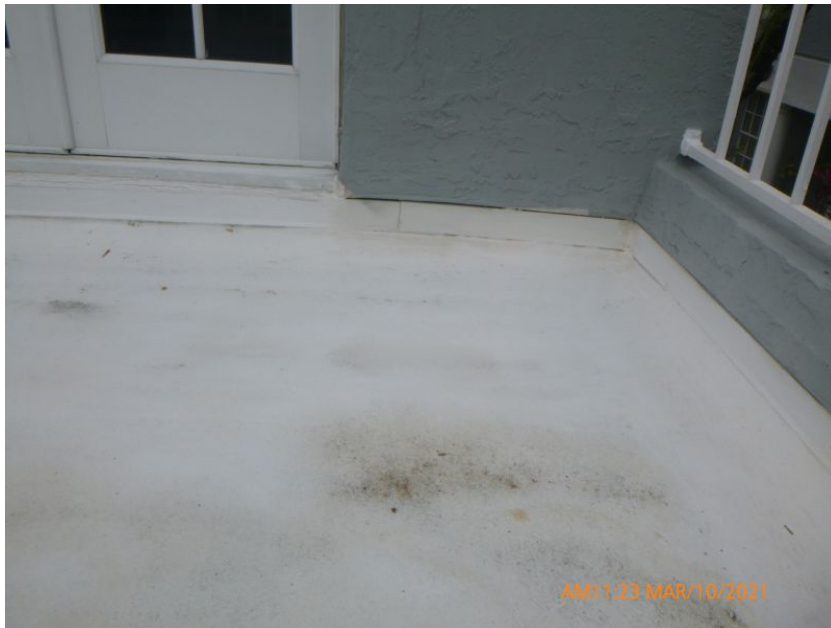
Built-Up/Rolled Asphalt Roof Covering
