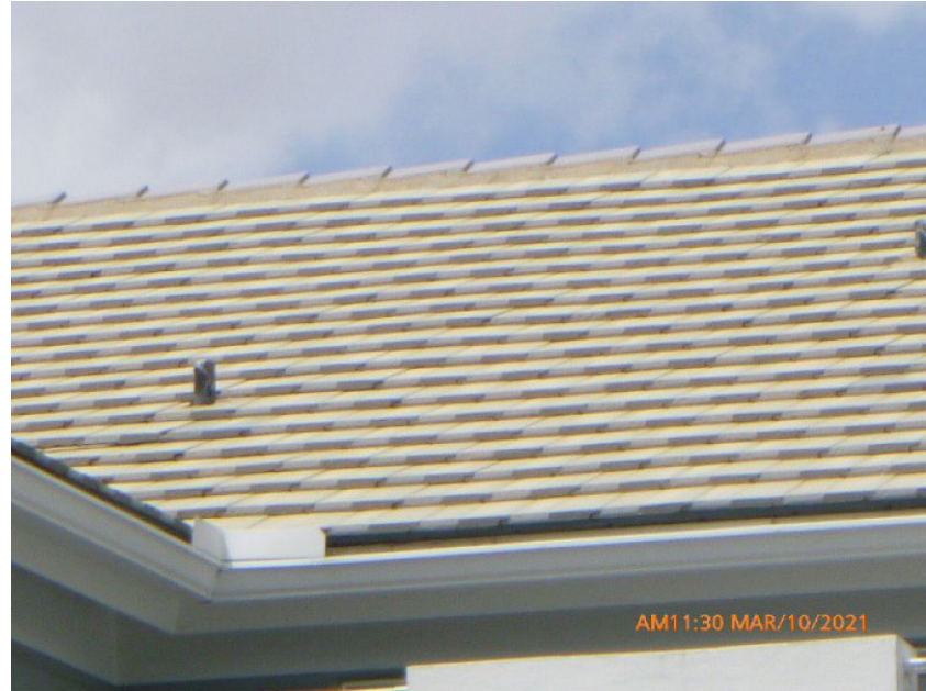
Concrete/Clay Tile Roof Covering
