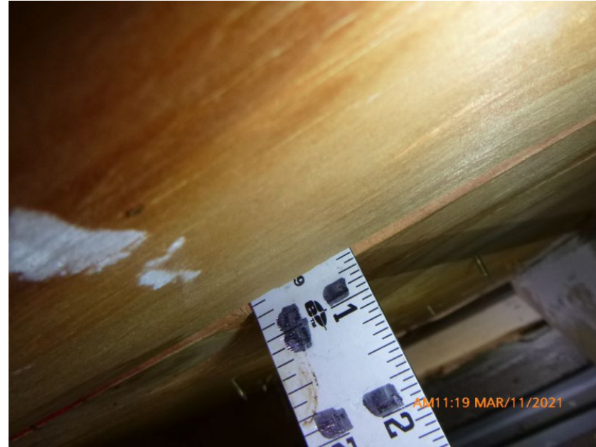
1 9/32" Deck Thickness Confirmed
