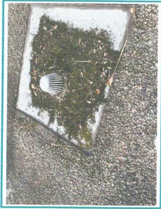
9. Interior drain clogged with vegetation/algae, clear out
