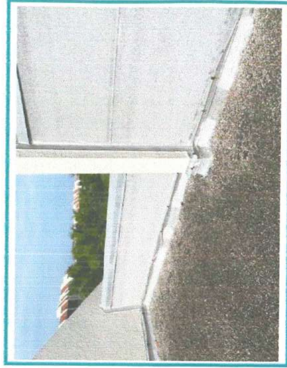
12. View of typical flashed parapet detail, well maintained
