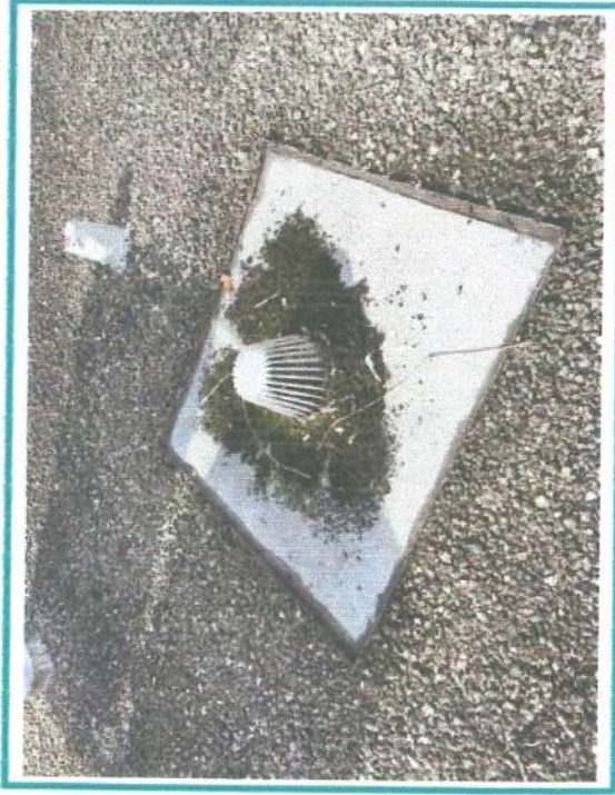
13 Interior drain hampered with algae/debris, clear out
