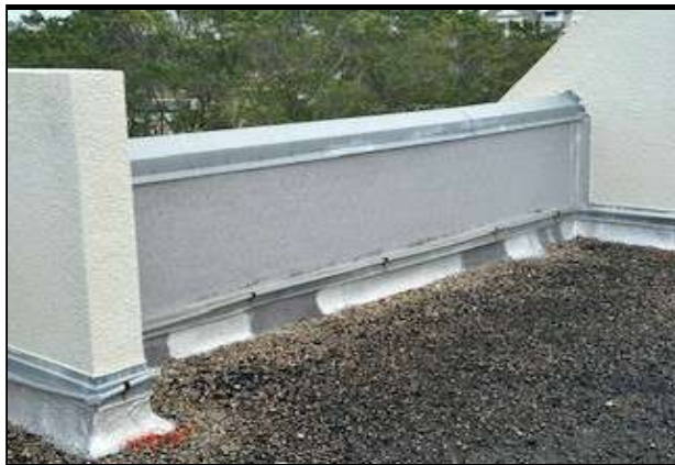
TYPICAL PARAPET WALLS BETWEEN MANSARD ENCLOSURES
