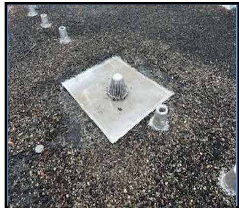
TYPICAL ROOF DRAIN
