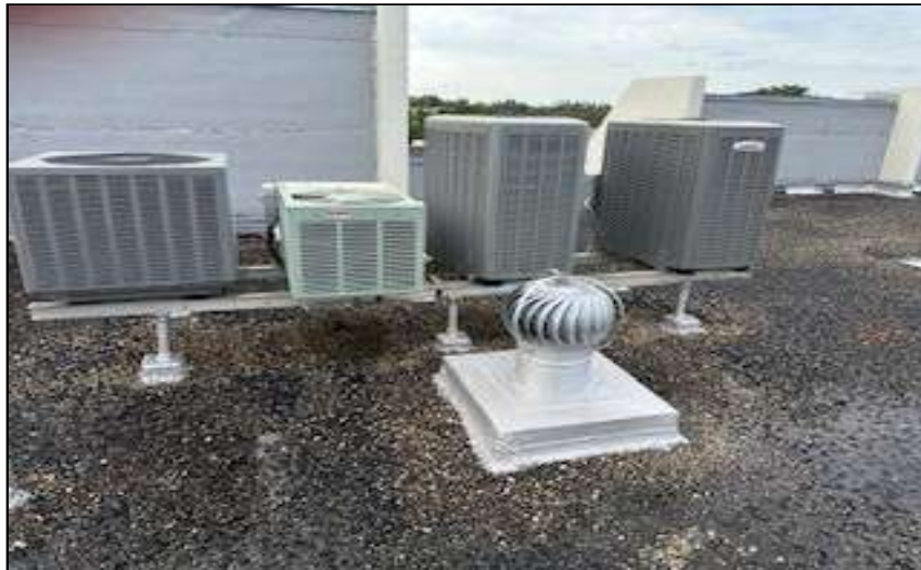
TYPICAL PLATFORM ELEVATED AIR CONDITIONING UNITS AND ROOF VENT
