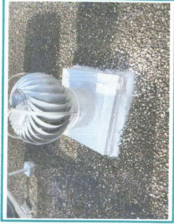
14 View of typical ventilator curb detail, well maintained
