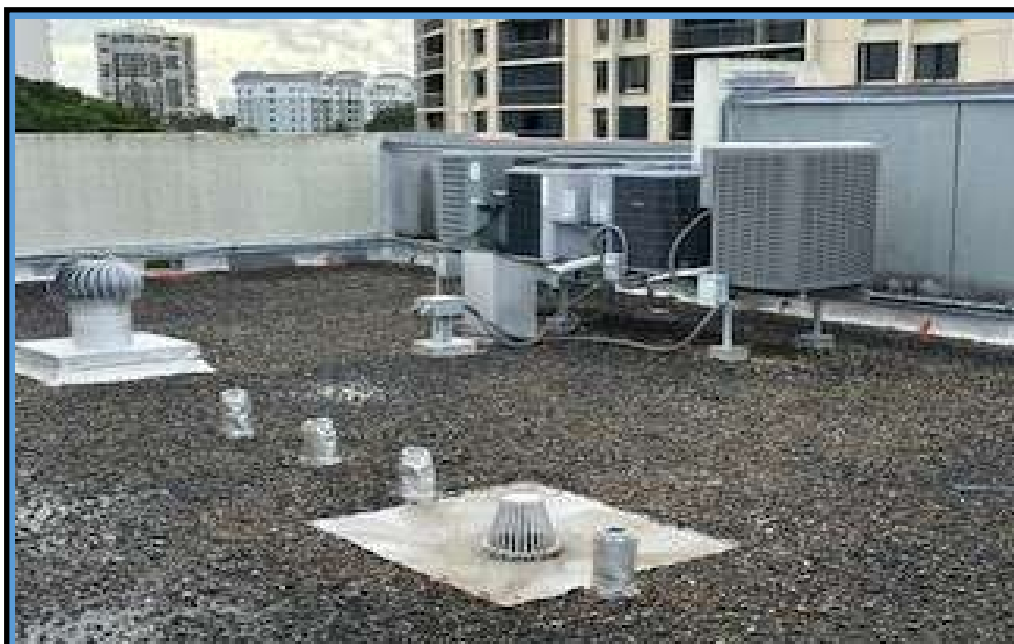
ROOF VENTS & A/C UNITS ON BUILT-UP GRAVEL ROOF
