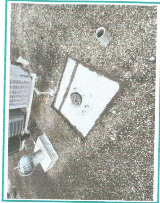
12. View of typical interior drain detail, boarder needs coating
