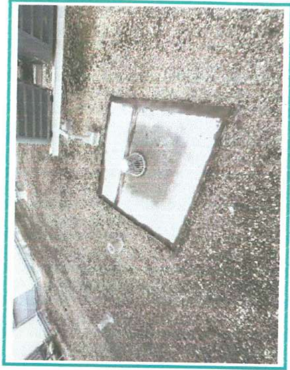
10. View of typical interior drain detail, boarder needs coating
