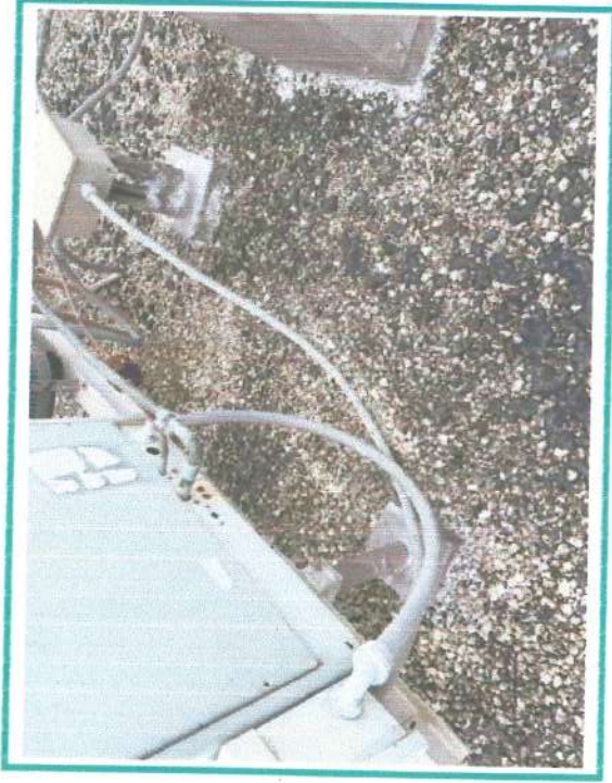
13 Typical penetration pitch pan detail, properly filled, coated
