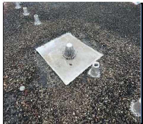
TYPICAL ROOF DRAIN
