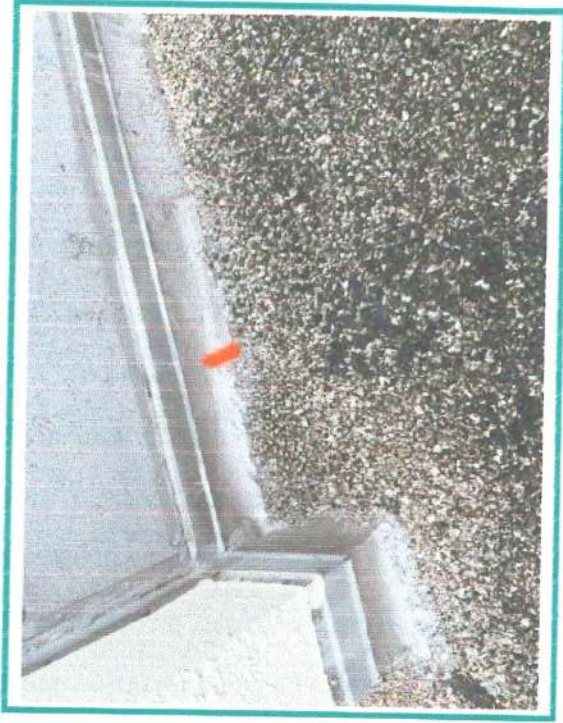
14 View of typical termination base detail, well maintained
