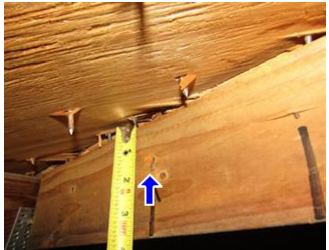
Roof to Deck Connection - 8D Nailing
