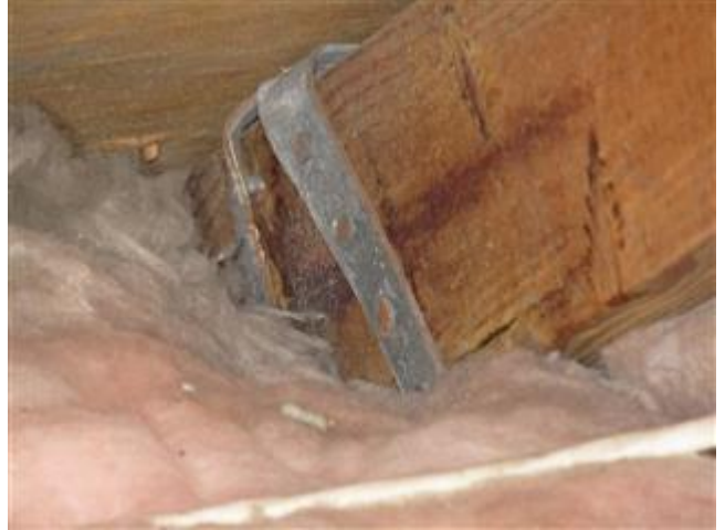
Roof to Wall Connection - Double Straps (Backside)
