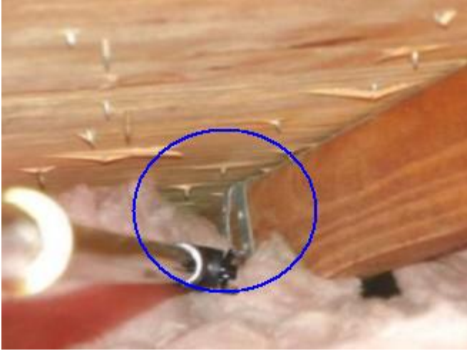
Roof to Wall Connection - Double Straps
