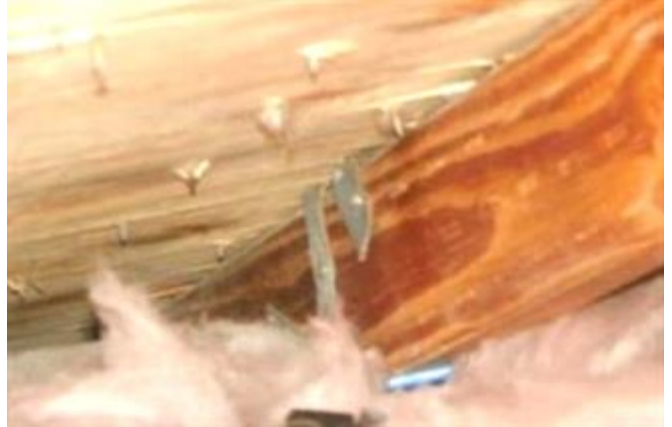
Roof to Wall Connection - Double Straps
