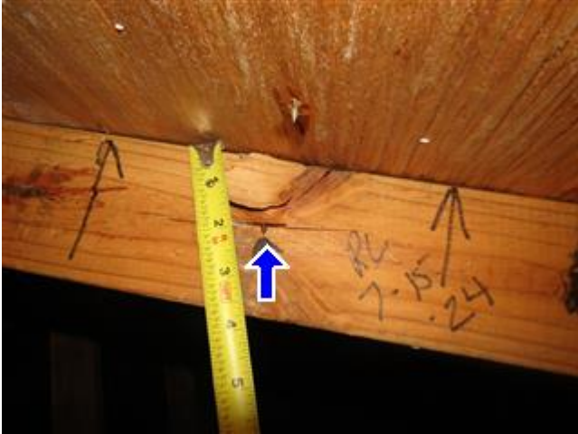
Roof to Deck Connection - 8D Nailing
