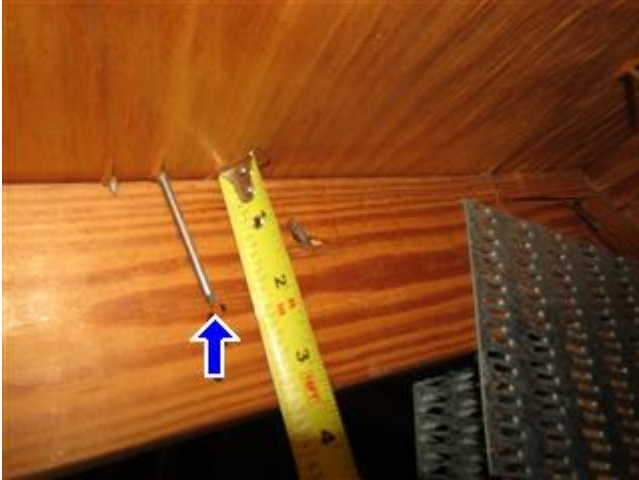
Roof to Deck Connection - 8D Nailing
