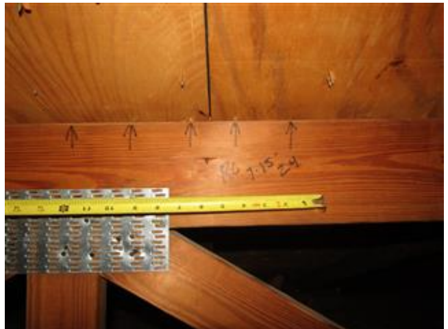
Roof to Deck Connection
