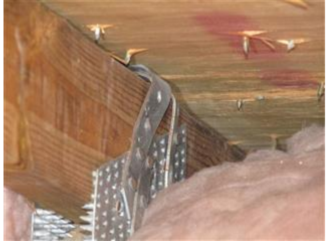
Roof to Wall Connection - Double Straps
