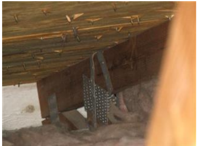
Roof to Wall Connection - Straps
