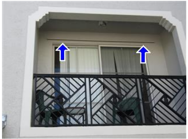
Hurricane Shutter Hardware - Glass Doors
