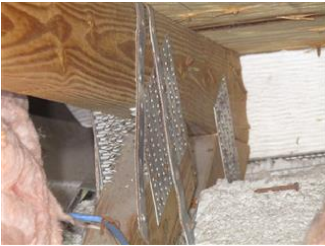
Roof to Wall Connection - Double Straps (Backside)
