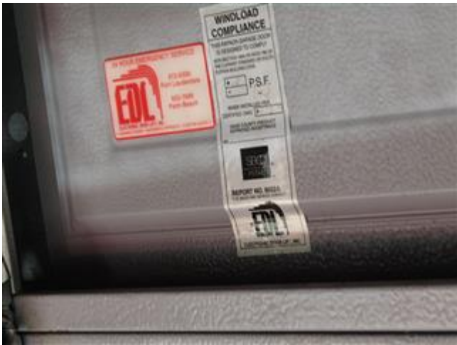
Hurricane Impact Garage Doors Verification
