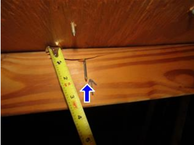
Roof to Deck Connection - 8D Nailing
