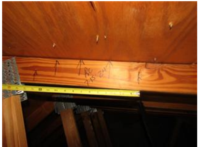
Roof to Deck Connection
