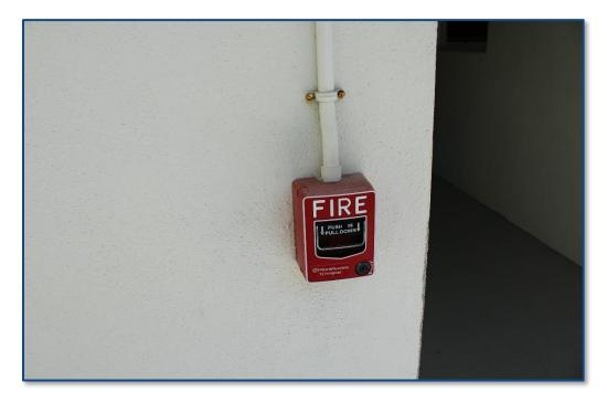
Photograph No. 14: Common area fire alarm switch.
