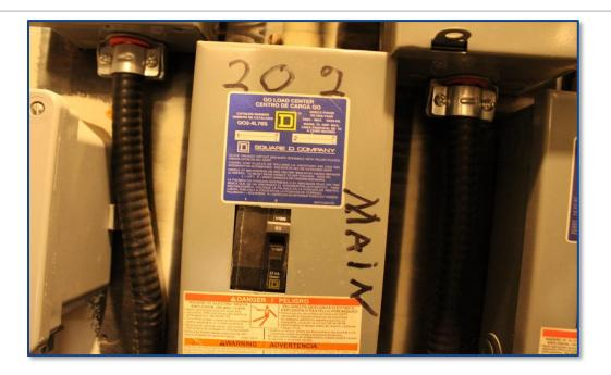
Photograph No. 19: Main switch for individual units.
